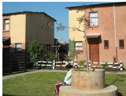
Figure 3: Two-storey semi-detached units in Sakhasonke with small neighbourhood space in-between the units
