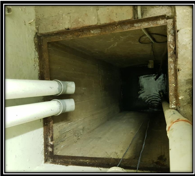
Figure 6A: Sump pump
