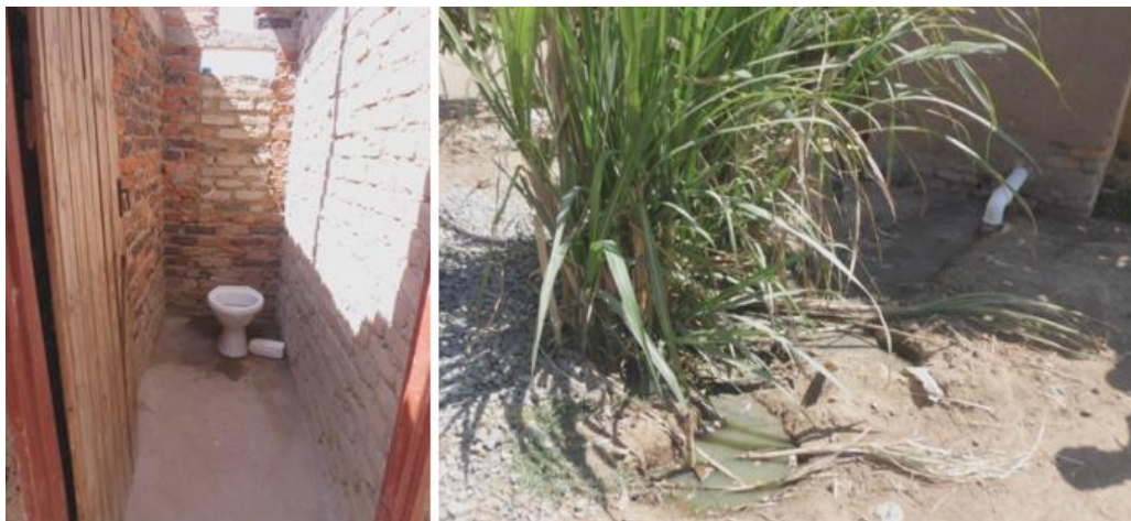
Figure 7.16 On the left, a sanitation facility on one of the stands showing the interior with only a seat but no water tank to use for flushing and on the right, showing raw sewage flowing to the outside
