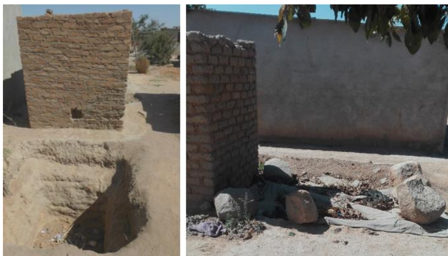
Figure 7.17 On the left, showing a toilet under construction with a hole to contain the excreta, and on the right, the hole is temporarily covered by plastic or other materials
