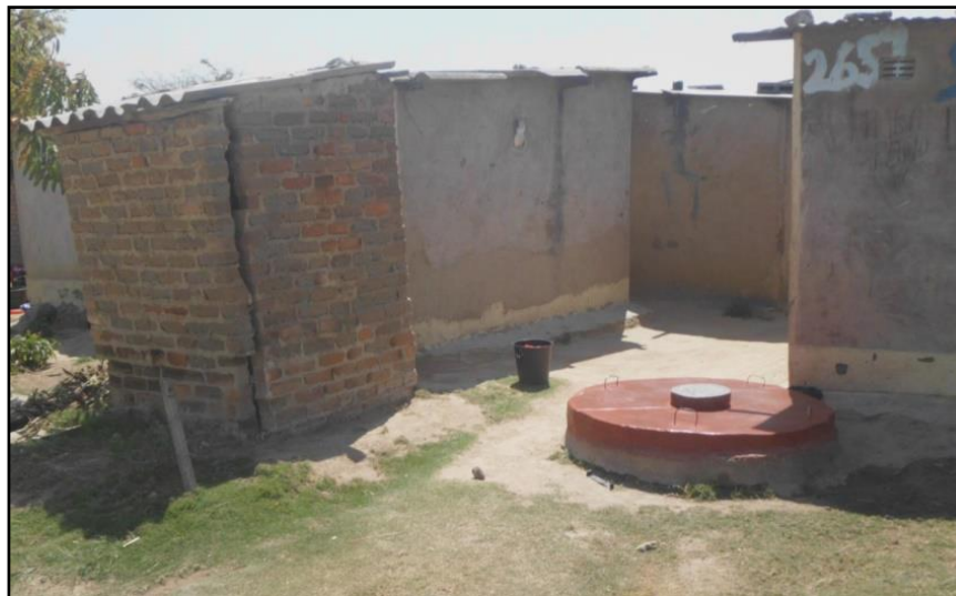
Figure 7.12 The close proximity of a pit latrine (on the left with the cracked wall) and a shallow well on the right
