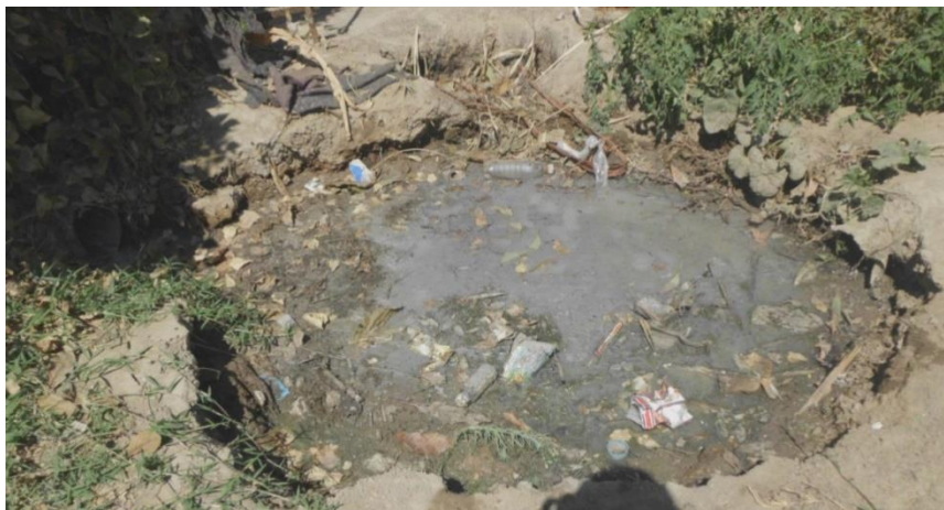
Figure 7.19 Sewage a pit filled up with faecal matter exposed to the surface
