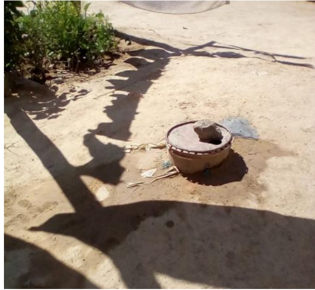
Figure 7.7: Shallow wells which are left open and or has a lid to cover it, referred to as ‘protected wells’
