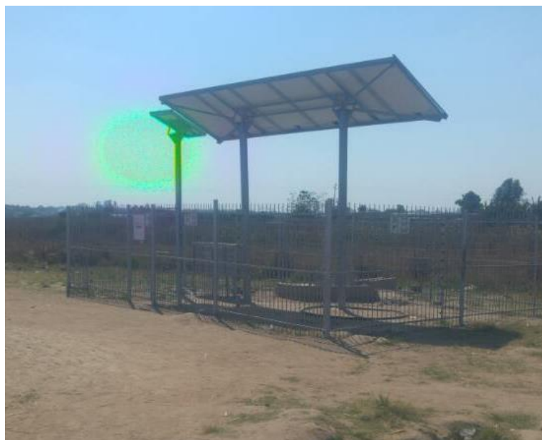
Figure 7.5 The solar system which powers the borehole supplying water to the school under construction in Hopley
