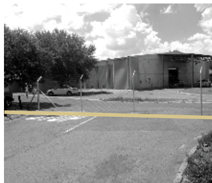
Figure 131: Road closed off with fence on north side of site
