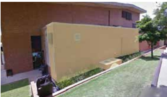
Figure 228: Location of services on southern facade (Googleearth, 2016: online).
