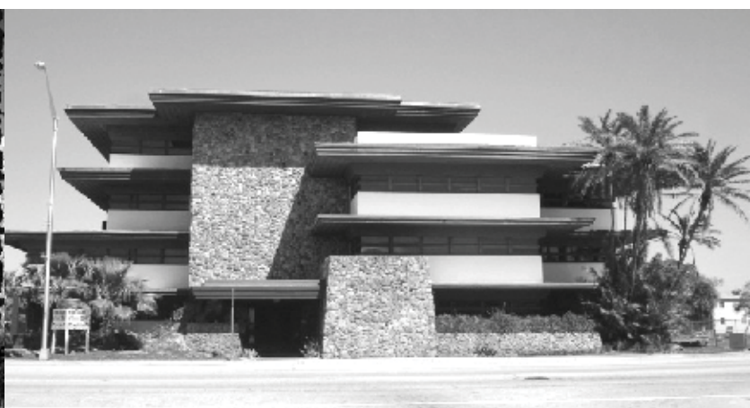
Figure 145: Research tower by Frank Lloyd Wright, and example of a building that stretches beyond its edges. (Lengkapku, 2015: online)
