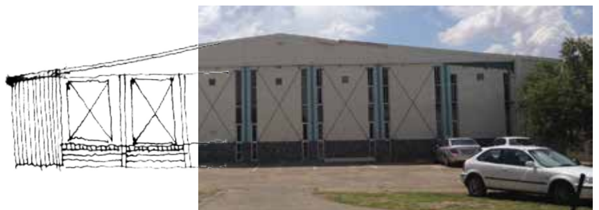
Figure 217: External bracing seen in surrounding buildings
