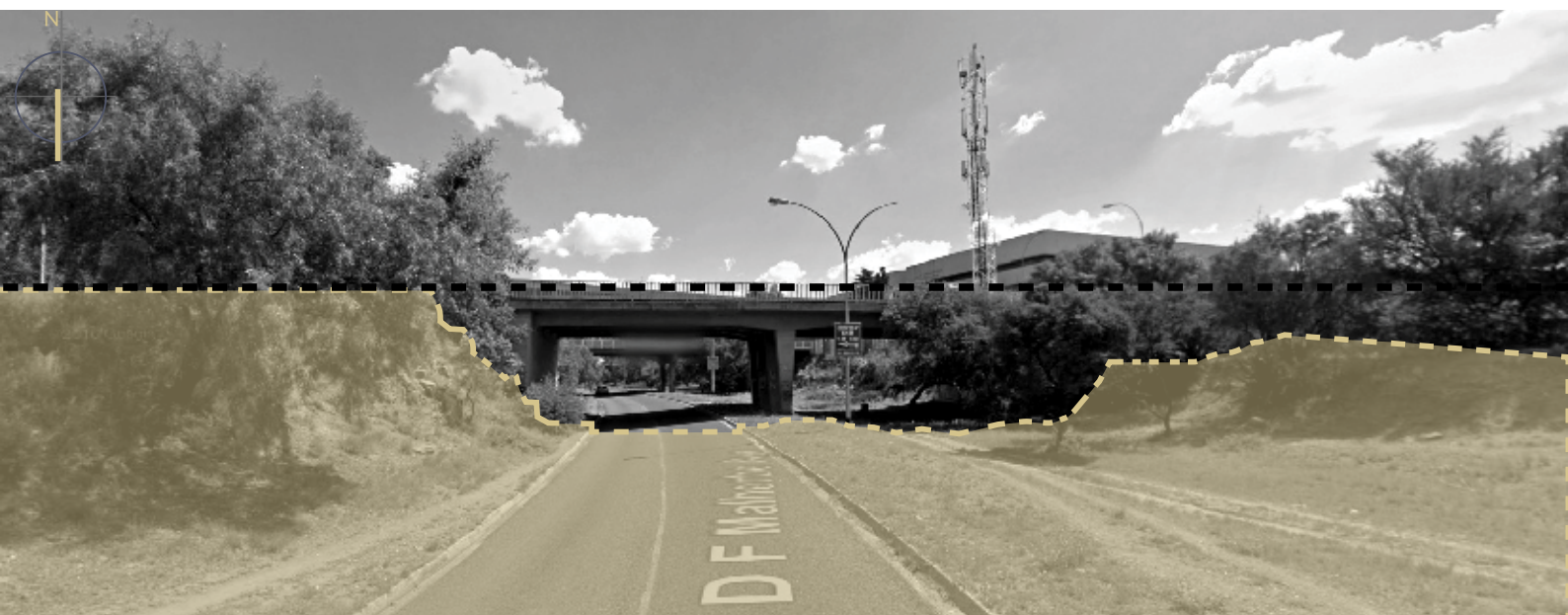
Figure 36: Carving process as seen on site from northern elevation
