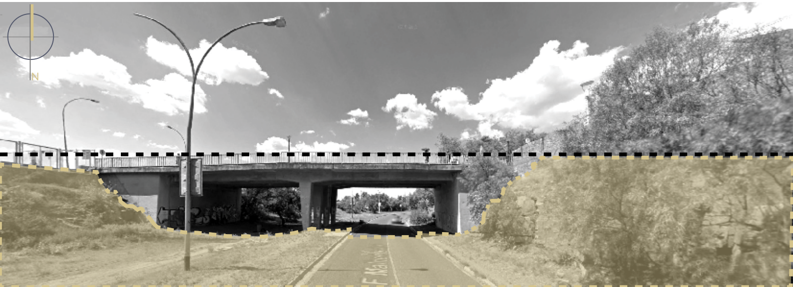
Figure 35: Carving process as seen on site from southern elevation
