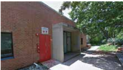
Figure 230: Fire door on southern facade of building (Googleearth, 2016:online).
