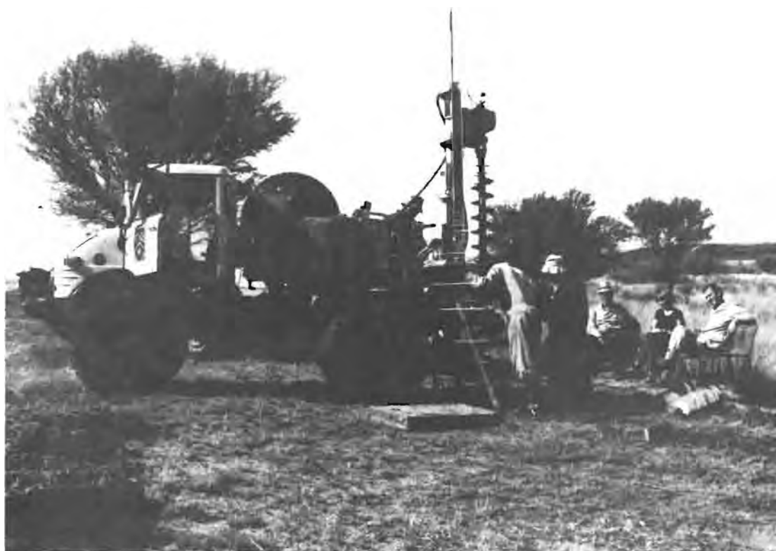
The mobile drill of the Geological Survey, Pretoria has lifted a column of sediment at the Florisbad swamp. The sediments are being recorded and sampled.
