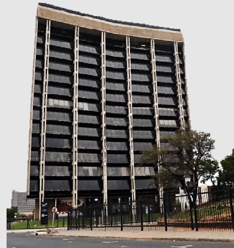
Figure 40: Current status of the Harry Oppenheimer House (Kimberly City Portal, 2022: online).
