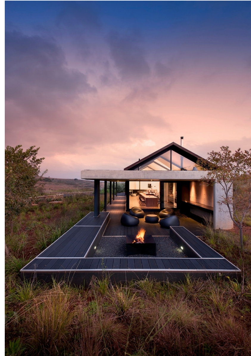
Figure 134: Side perspective of the building showcasing the effortless outdoor and indoor transition (ArchDaily, 2022: online).
