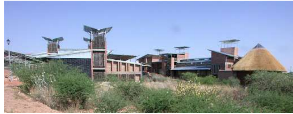
Fig. 166- The Habitat Research and Development Center (Nina Maritz Architects, 2004: online)
