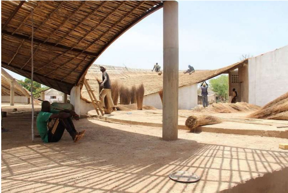
Fig. 186- Senegal cultural center during construction (Author, 2021)
