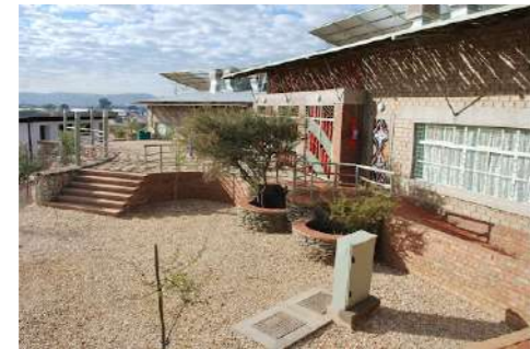
Fig **. The Habitat Research and Development Center (Nina Maritz Architects, 2004: online)
