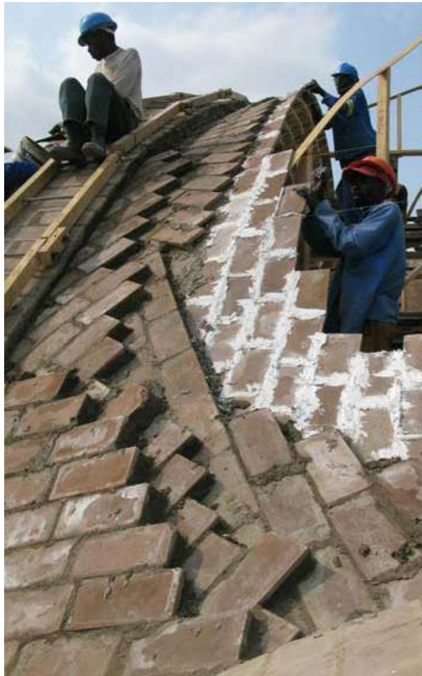
Fig.196- Roof during construction (Selkou, n.d.: website)
