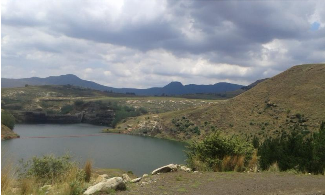
Figure 4.2: Muela Dam, from which water is transferred to South Africa
