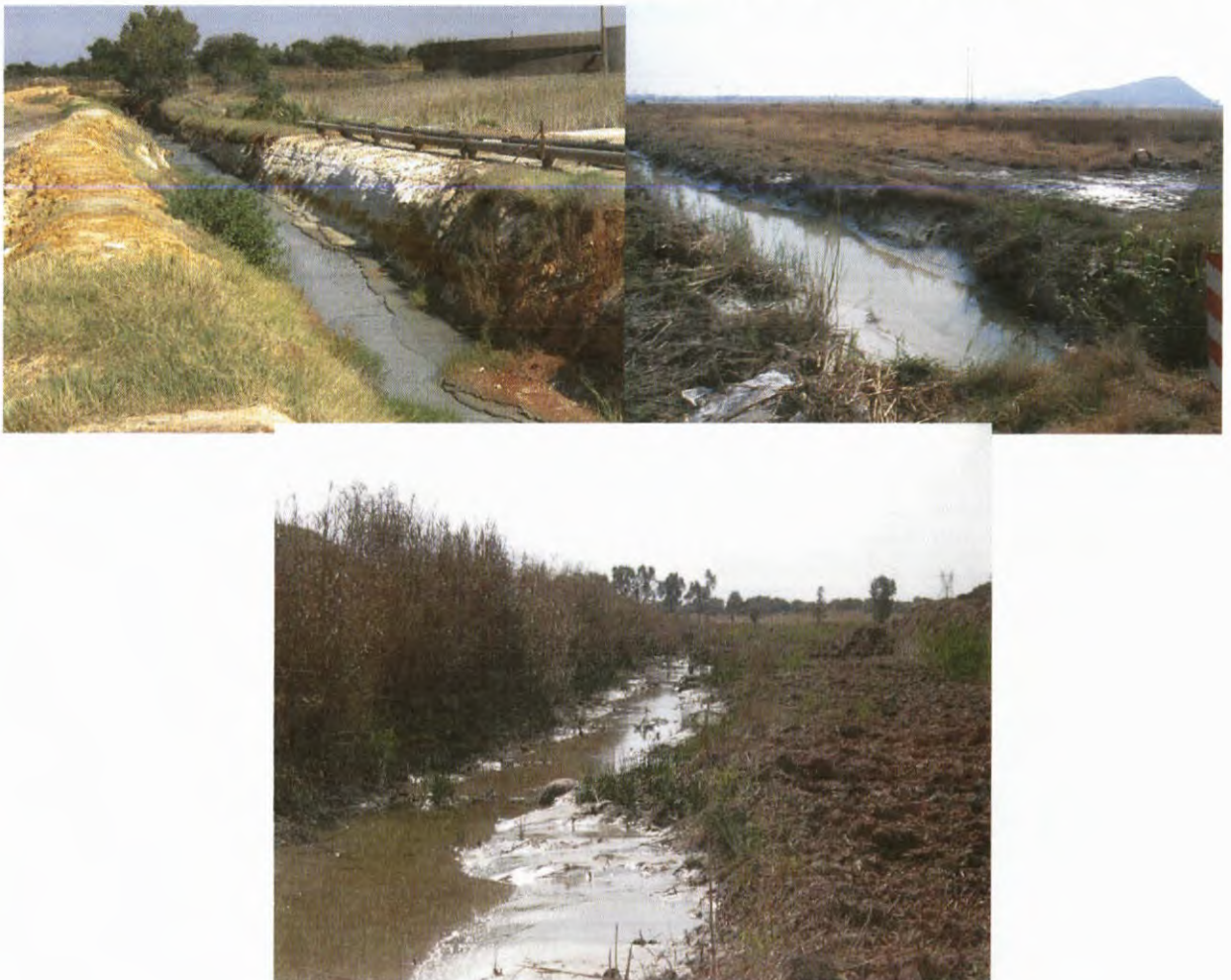
Figure 7: Photos of typical earth effluent trenches
