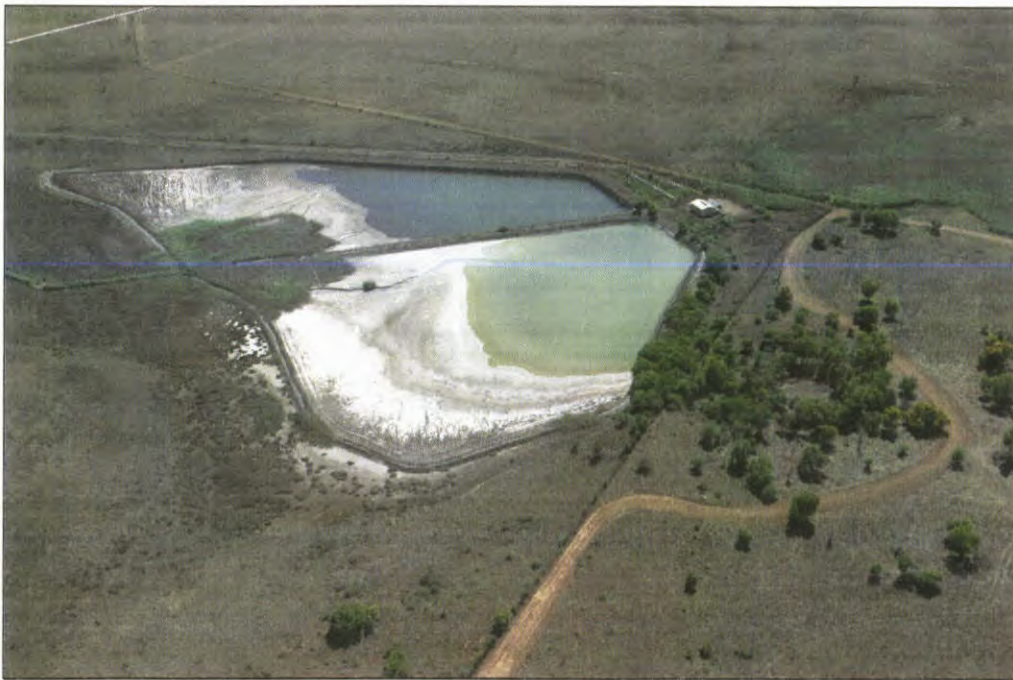
Figure 8: Photo of Bokkamp Dam RWD within the investigation area
