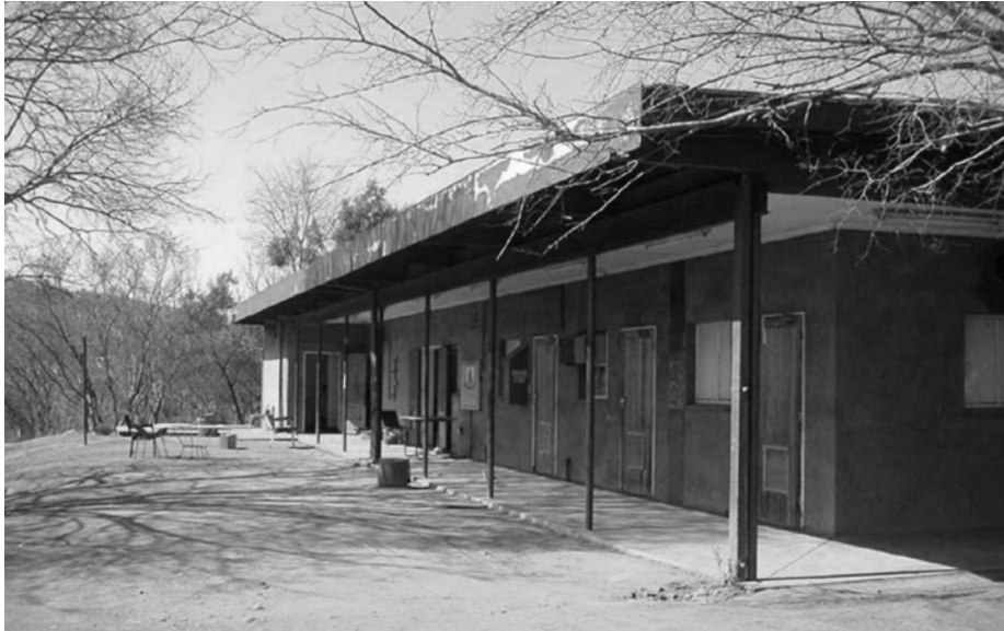
Figure 67: Outside of Building 5300 (Albright and Stricker, 2016).
