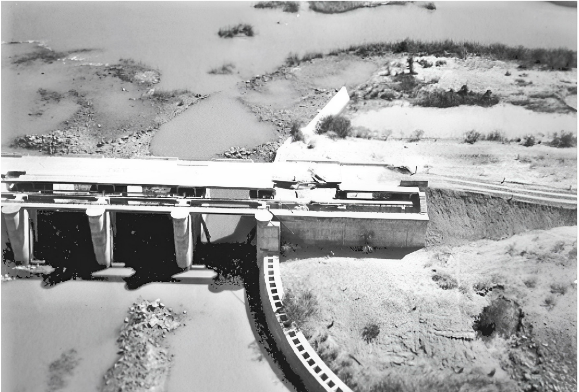
Figure 13: Targeted and bombed bridge in Angola showing structure physically changed through conflict (Venter, 2019).
