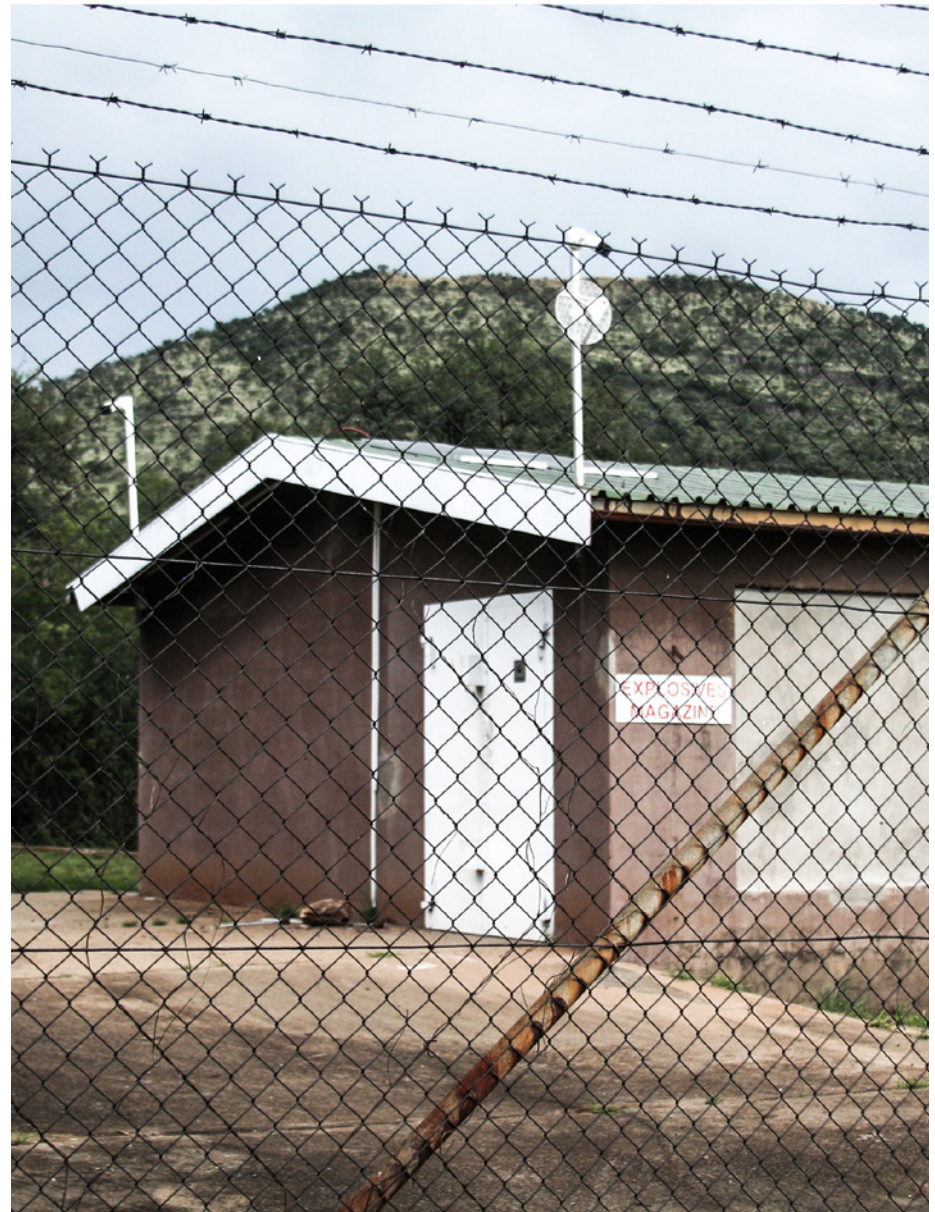
Figure 69: The heavy walls of the magazine (author, 2023).
