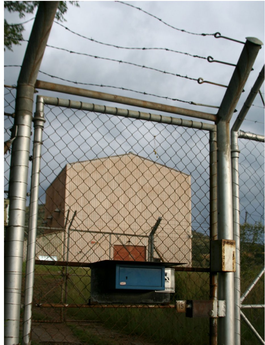
Figure 4: The restricted site, the first glimpse, building 5000 (author, 2023).
