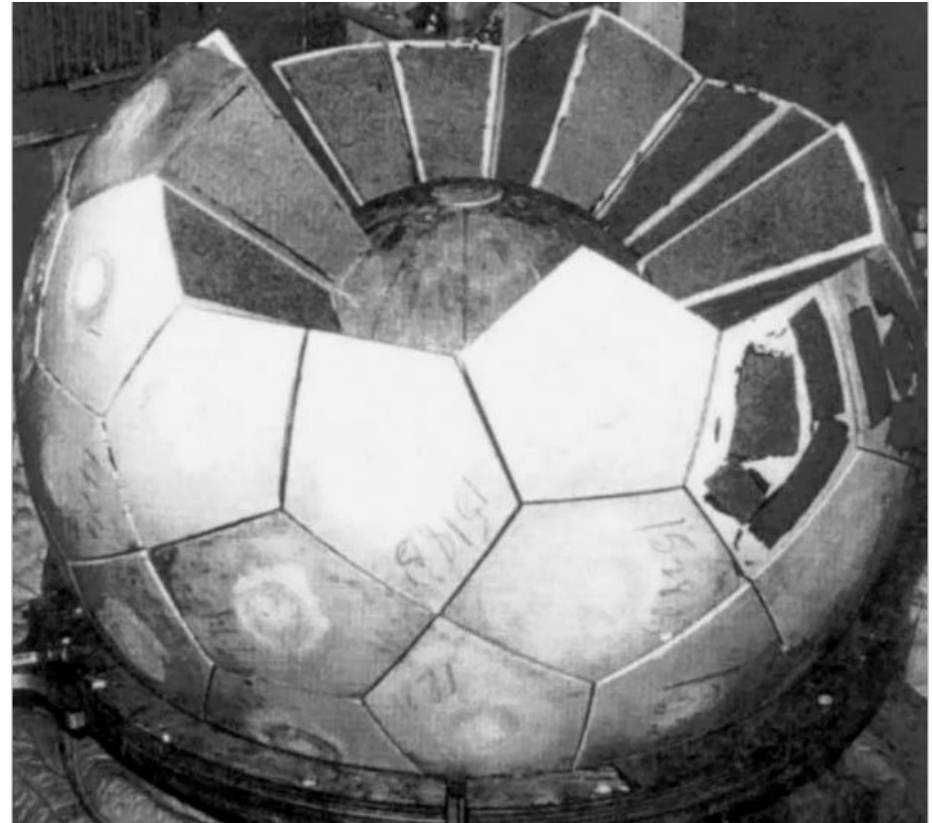
Figure 18: An implosion-type assembly at Los Alamos and later used in the first nuclear explosion, the Trinity Test (AHF, 2017).
