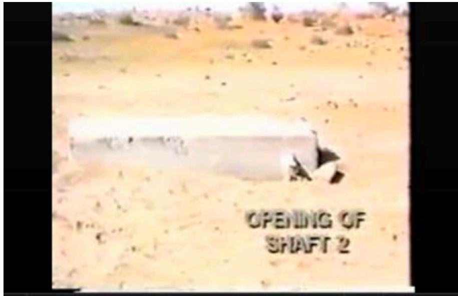
Figure 26: Shaft 2, before reopening (ISIS, 2018).
