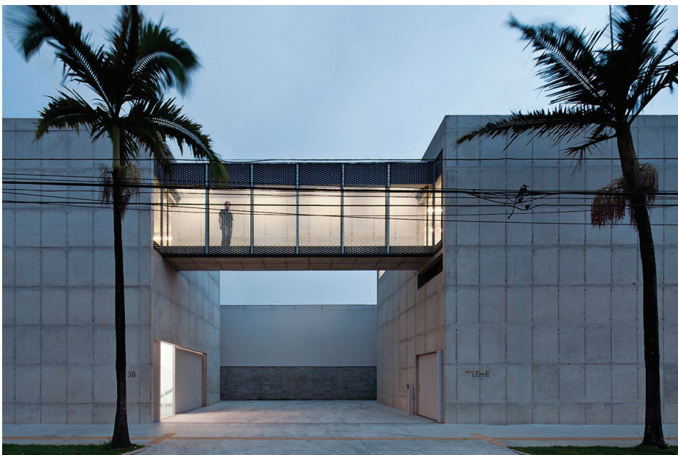
FIGURE 114 Street view of the New Leme Gallery, the porous footbridge connecting the two masses (Archdaily, 2013: online).
