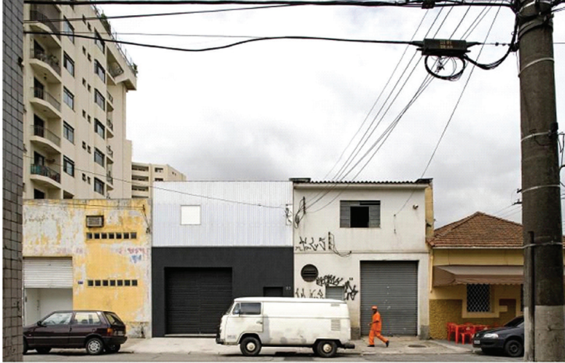
FIGURE 111 Street view of the Leme Studio. The facade borrowed from the context (Phaidon Atlas, 2006: online).
