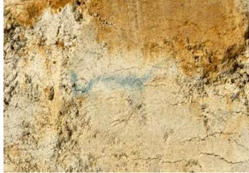
Figure 8.2: Blue staining found on the tailings dam in Welkom, South Africa. This is believed to be an iron-cyanide compound and is ~3 cm in length.
