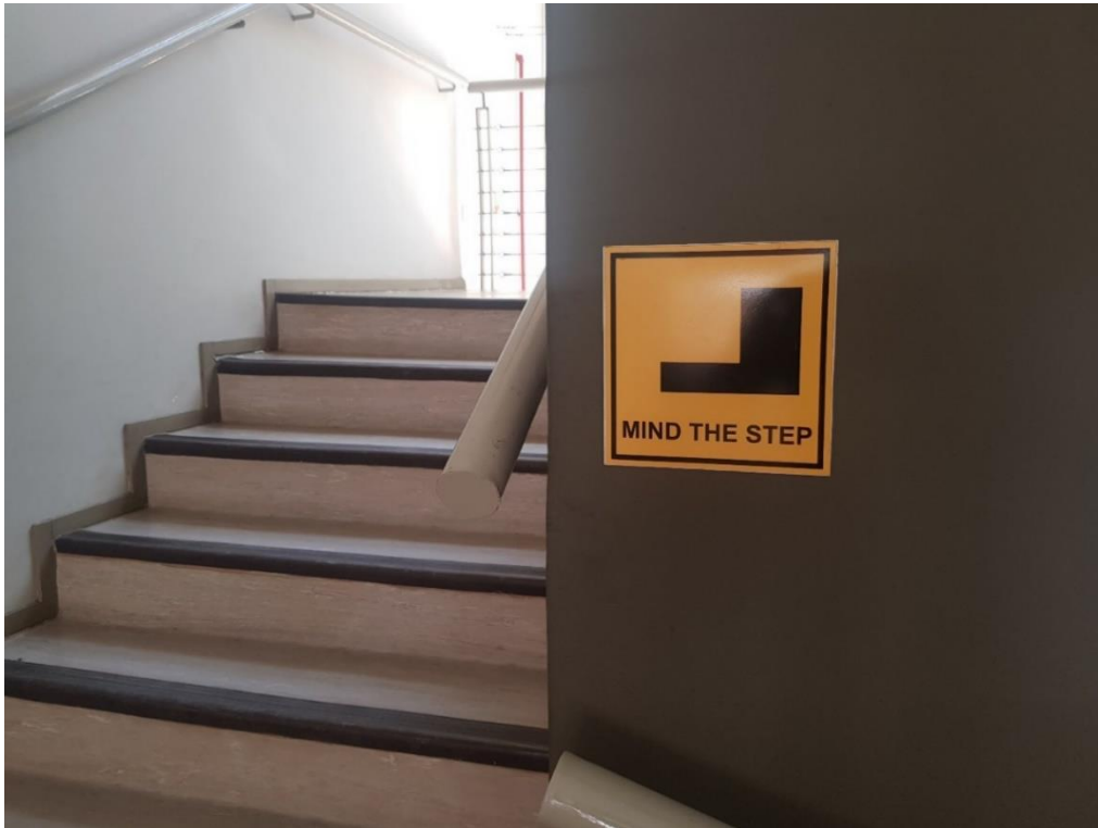
Figure 4.8 Stairs caution sign in the chemistry building
