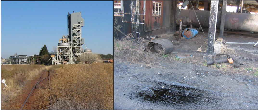
**Figure 5-56: View of the decommissioned gasworks, with spillage from tar loading tanks, still visible.**
