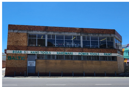
Figure 25: Baltic Timber hardware store, not conservation worthy (Author, 2023)
