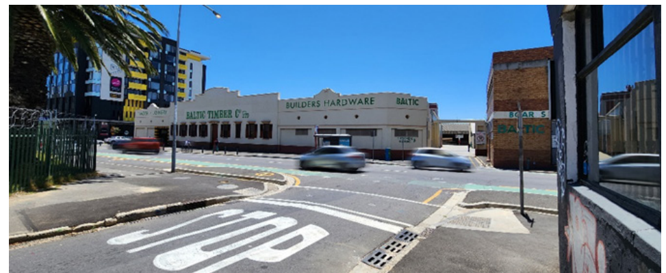
Figure 27: Photograph of main historic gable (Author, 2023)
