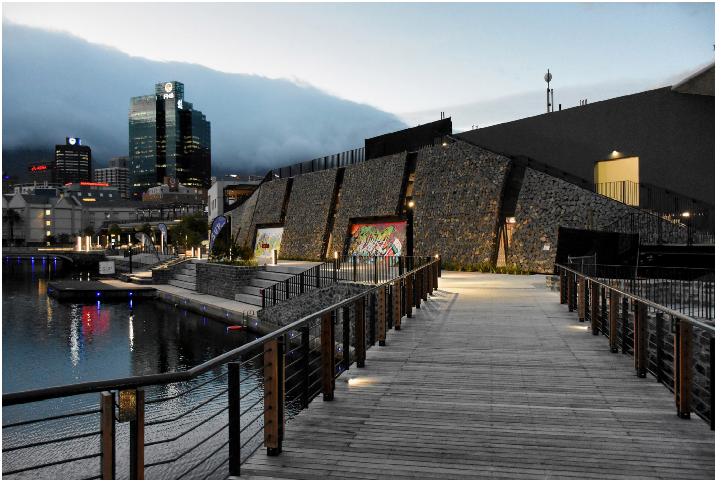
Figure 79: New building compliments and acknowledges the past (de Klee, 2019: online)
