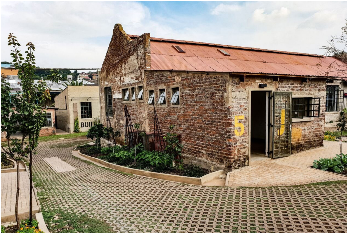
Figure 72: Material composition of buildings in Victoria Yards (Daffonchio Architects, 2018:online)
