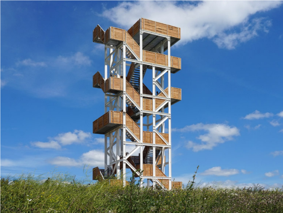
Figure 178: Viewing Tower Hoge Bergse Bos (Ateliereen Architecten, 2017: online).
