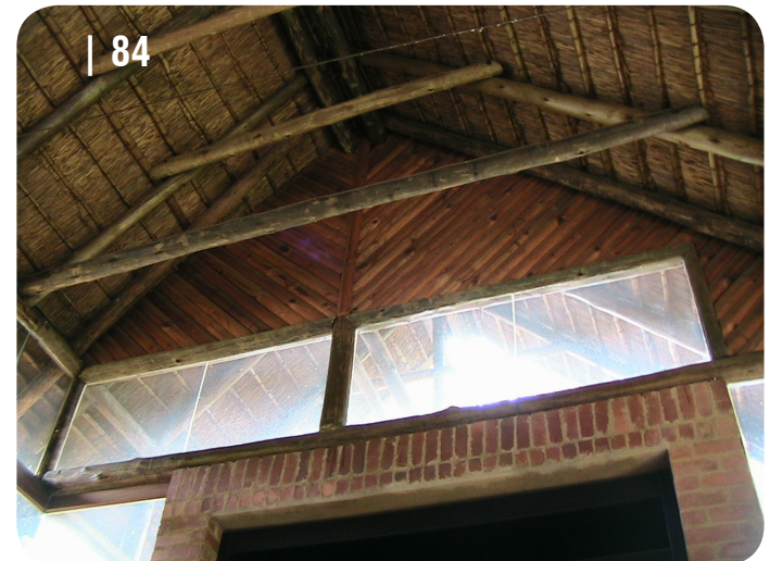
fig. 86 A groove is made in the gum-poles where glass panels are inserted flush against the timber and sealed with silicone.
