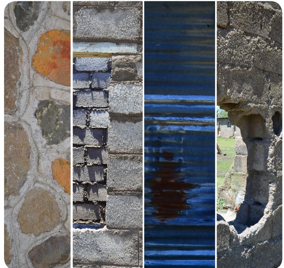
fig. 55 Textures regularly visible in Semonkong and Ha Lesala: stone, concrete block [ usually of bad quality cement ], corrugated iron.
