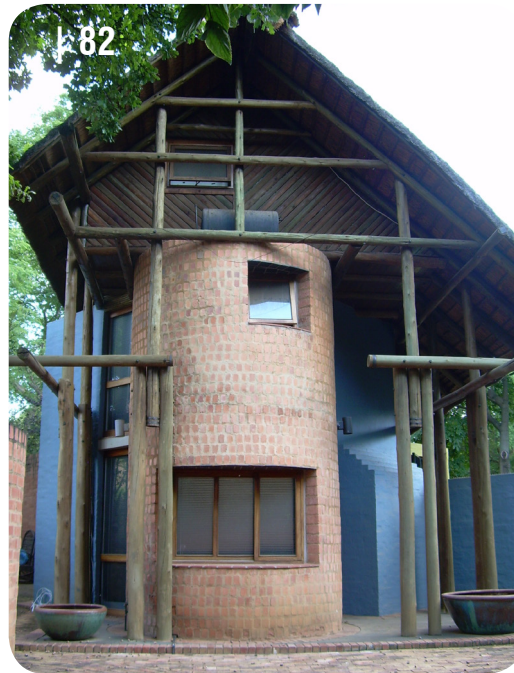
fig. 84 Structural system made up off gum-poles as tectonic framed structure to be filled in.
