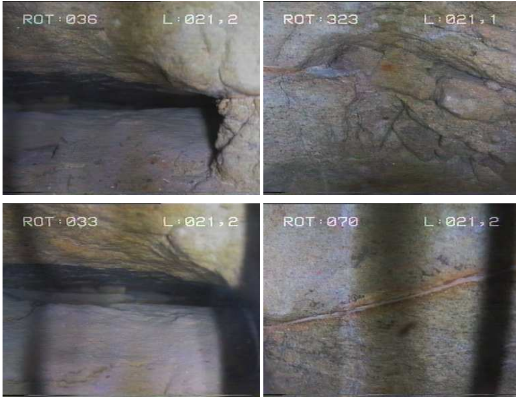
Figure 3-11 Borehole video camera observations in UO20. (Fracture zone).
