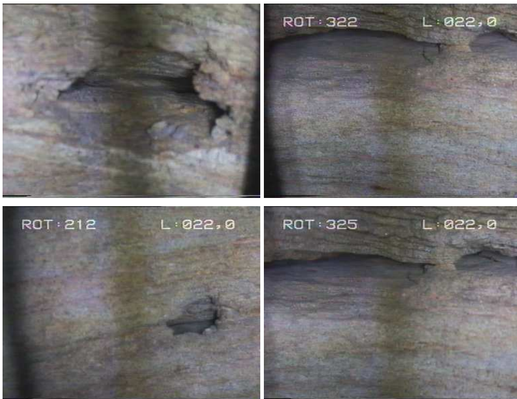
Figure 3-12 Borehole video camera observations in UO14. (Fracture zone).
