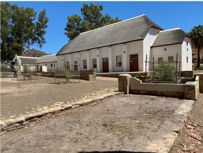
Figure 2.19: Town Hall built in 1981 (Author, 2022).
