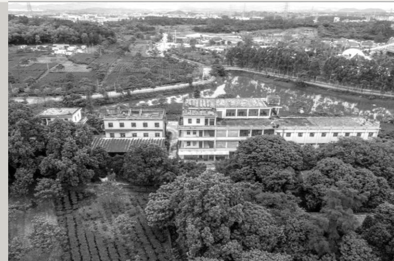
Figure 6.18: image of historic tea production factory (Shuangyu, 2020; online).
