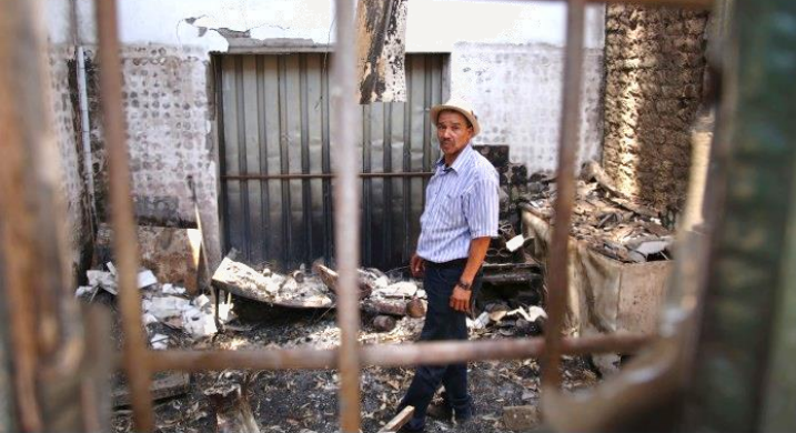
Figure 3.7: Barend Salomo, Managing Director of the Wupperthal Original Rooibos Co-Op, standing in a building damaged by the fire of 2018 (Isaacs, 2019: online).
