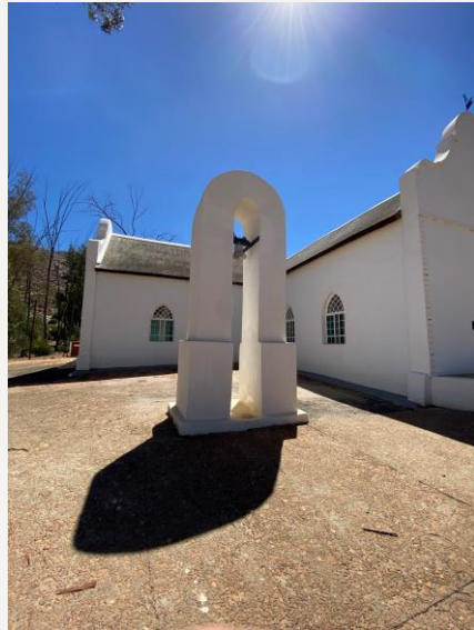
Figure 8.28: Bell tower (Author, 2022).
