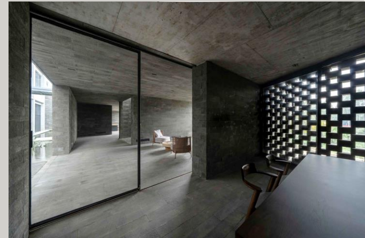
Figure 6.24: Light filtered through the granite podium and brises soleil details (Shuangyu, 2020: online).
