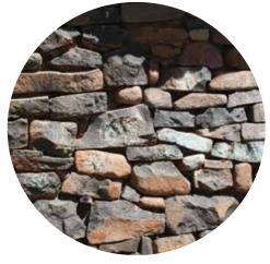
FIGURE 385: Local iron stone used to construct the birth place of James Moroka
