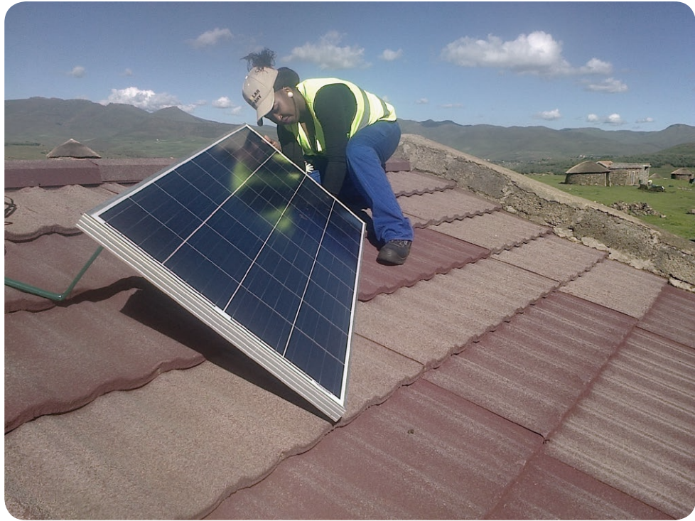
Solar panel installation in Semonkong (The Solar Company, 2019: online).
