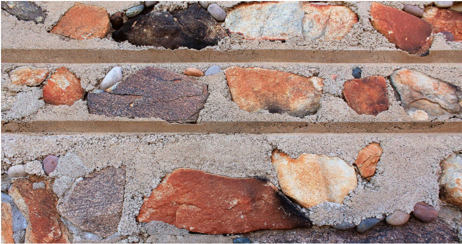
Figure 3.2.26: Desert masonry wall (Atlas of places 2019; online)
