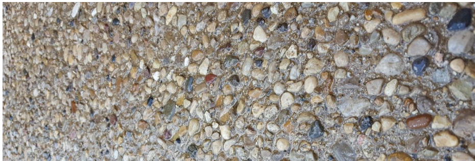
Figure 3.2.27: Exposed aggregate concrete to be used for exterior paveways
