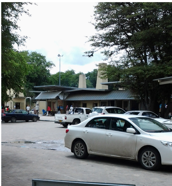
Figure 107: Market square, currently the parking by Mackintosh and Lautenbach Architects
