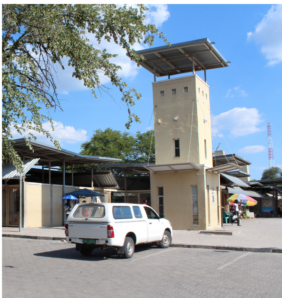
Figure 106: Market entrance from the north by Mackintosh and Lautenbach Architects
