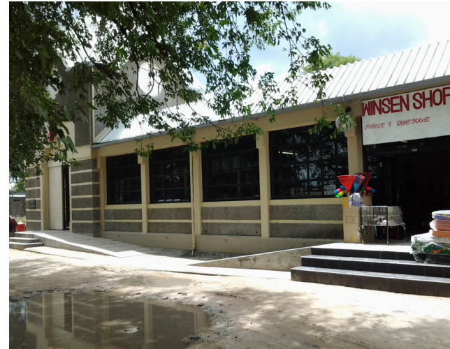
Figure 120: Post Office main entrance (far left) _ March 2015
