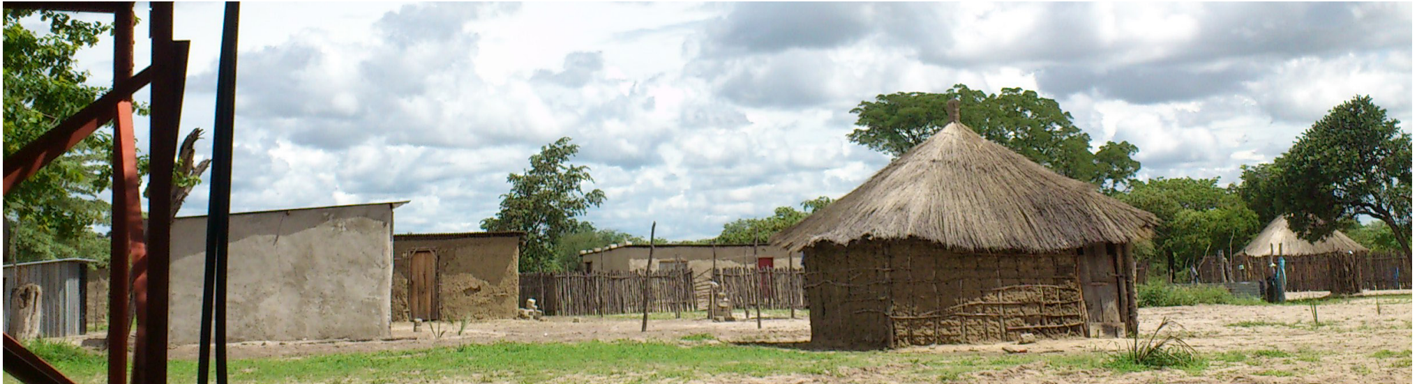
Figure 57: Habana village_ typical hut (foreground) and new hut house (background)
