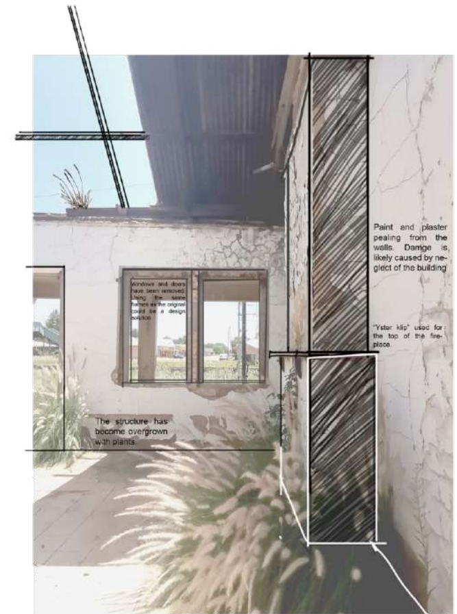
Fig 3.35: Image of interior of train station.
