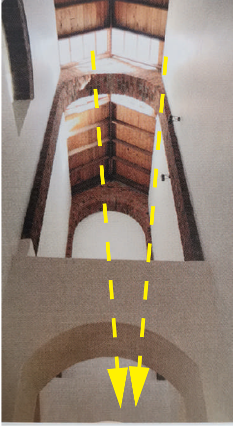
Fig 4.27: Image of Skylight flooding interior with light adapted by author (Herholdt, 2014: 275)
