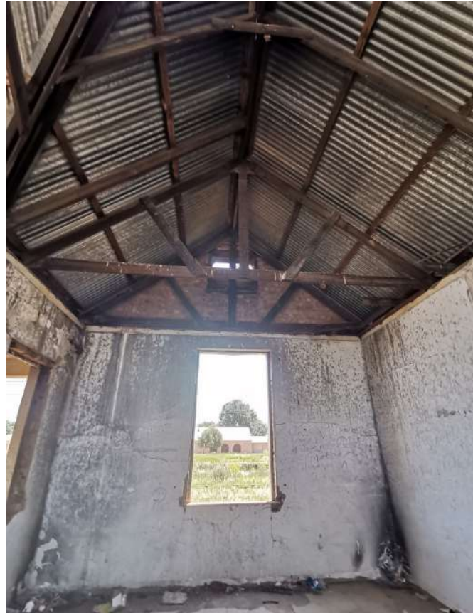
Fig 3.34: Image of interior of train station.
