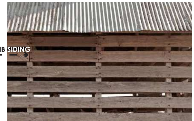
Fig 4.11: Barn exterior indicating materials (Crosby, 2015: online)
