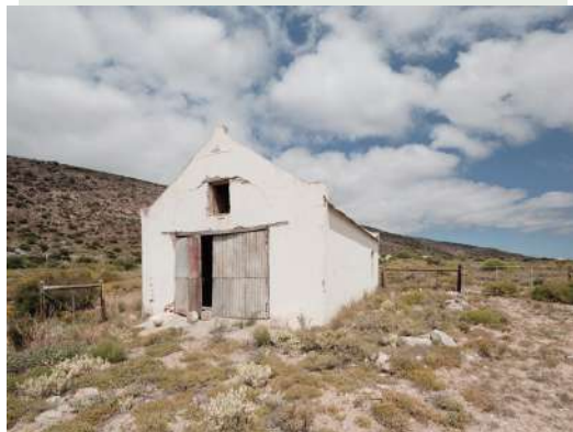
Fig 2.13: Photograph of Karoo Shed constructed with local materials (Schoeman: 2012, online)
