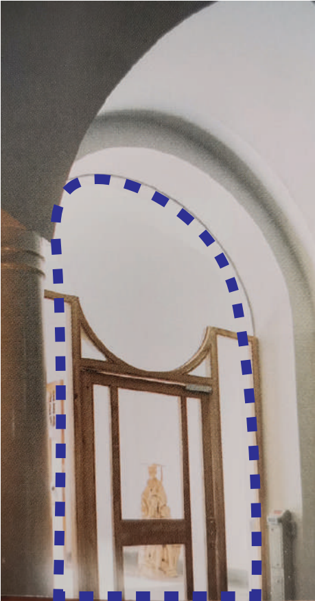
Fig 4.25: Photograph of entrance with light flooding into the interior, adapted by author (Herholdt, 2014: 275).
