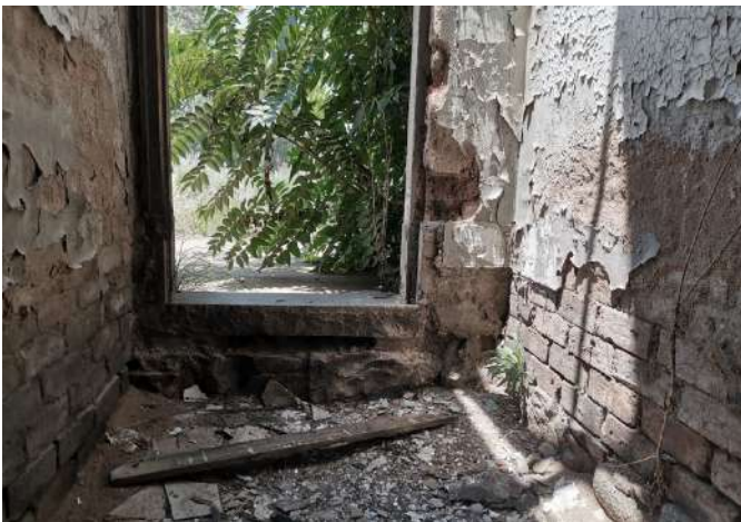
Fig 3.36: Photograph of ironstone foundation.
