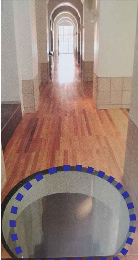
Fig 4.26: Image of skylight from first floor adapted by author (Herholdt, 2014: 275)
