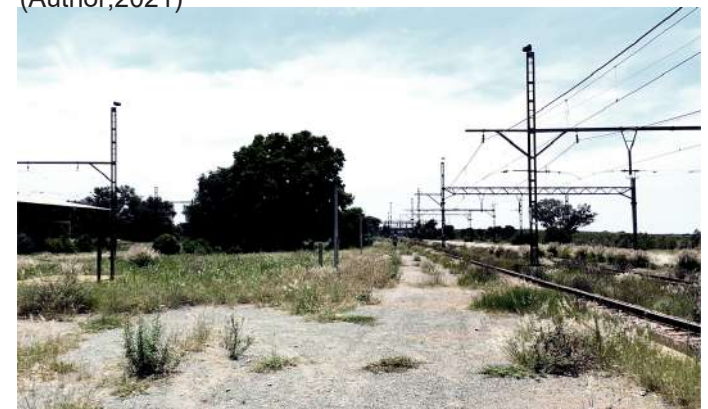
Figure 1.7: Image of railway lines (Author;2021)
