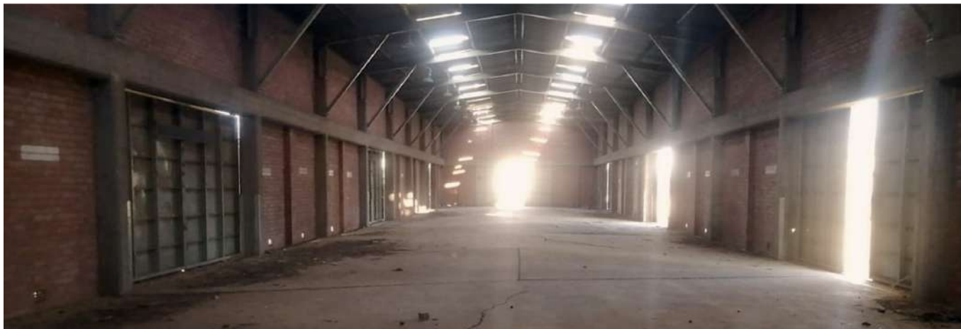
Fig 3.46: Interior of the shed.
