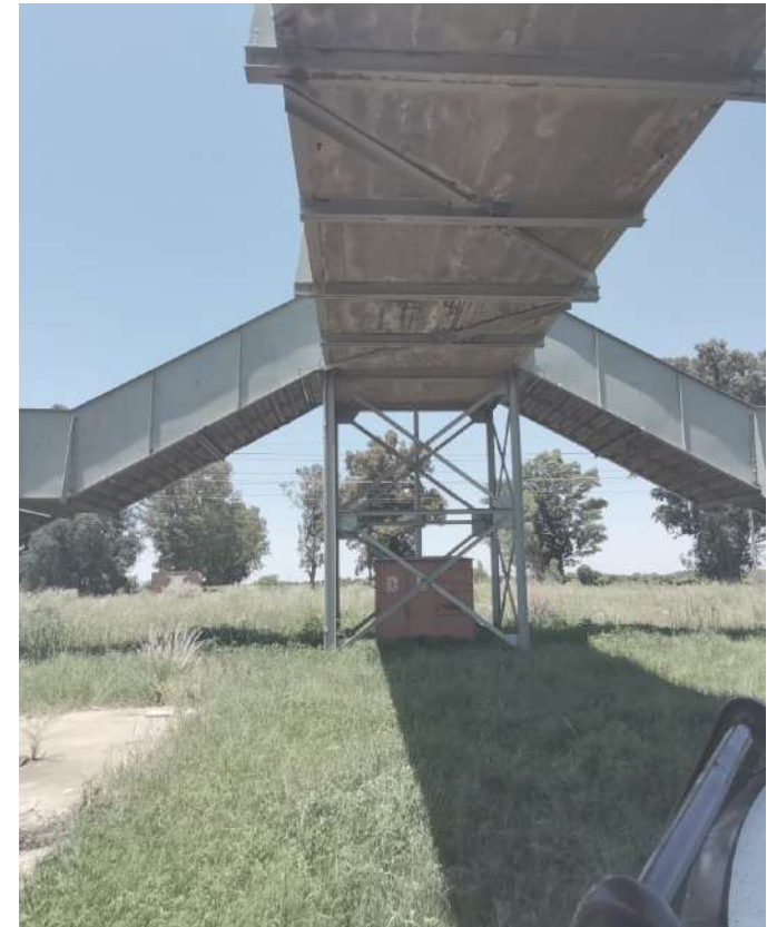
Fig 3.52: Image indicating power box underneath the bridge.
