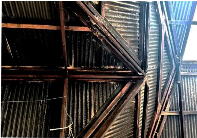
Fig 3.43: Photograph of the roof.
