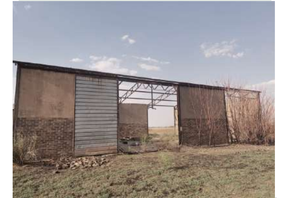
Fig 2.15: Photograph of farm shed in Makwassie district (Author: 2021)
