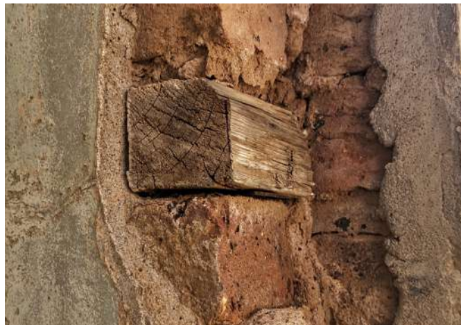
Fig 3.37: Timber window frame still visible in current structure
