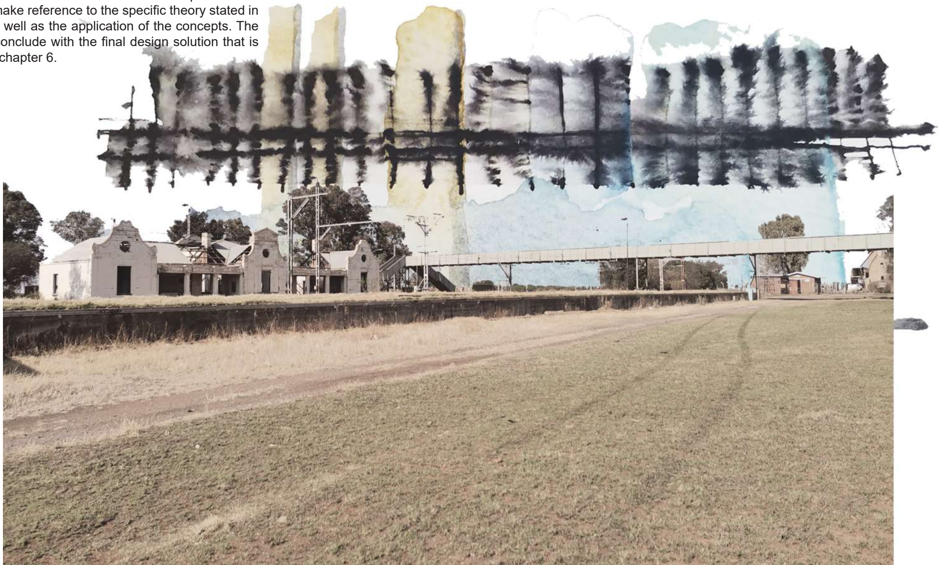
Fig 5.7: North elevation of Train Station
