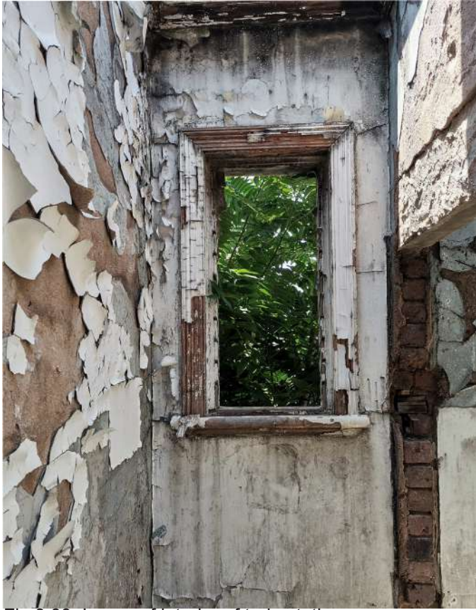
Fig 3.39: Image of interior of train station.
