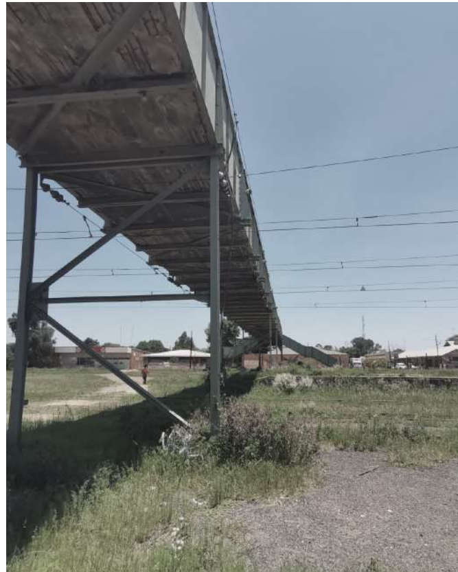
Fig 3.51: Image of the bridge.
