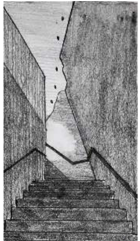
Fig 41. Staircase in Freedom Park building resembling a crevice in a boulder where light falls through.
