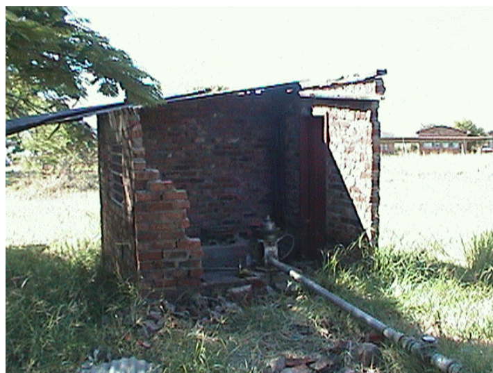
Figure 20 Borehole installation in the H12-region where bricks were taken away
