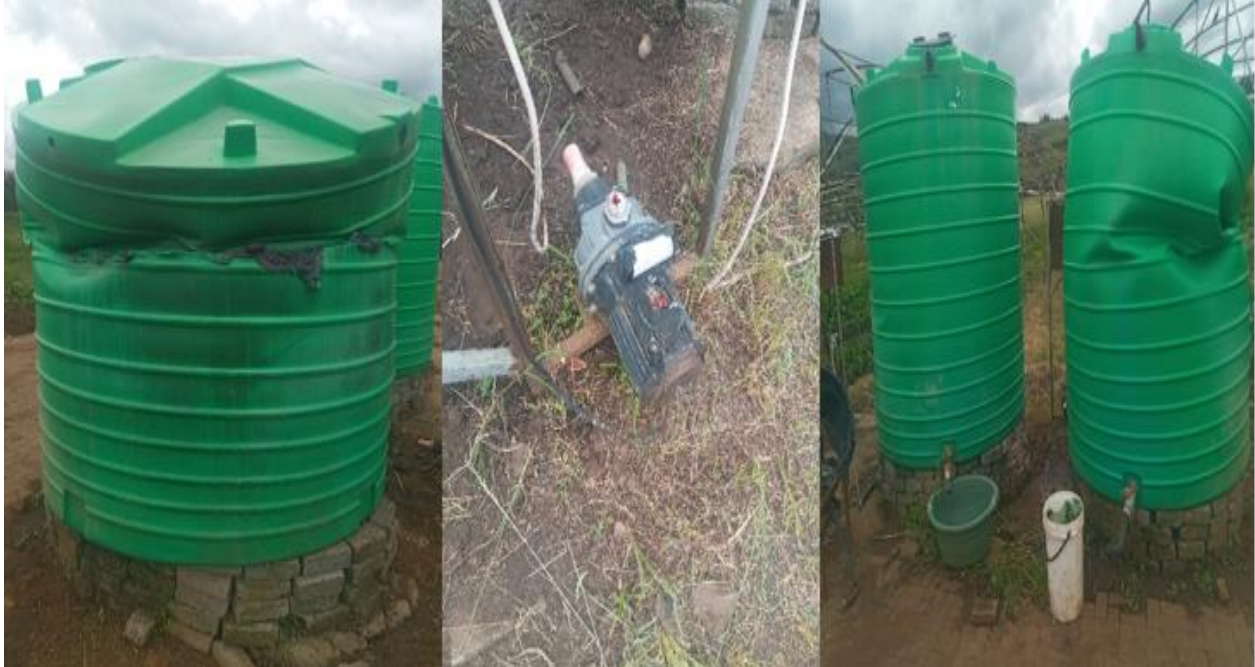
Figure 37: Project X's Water Pump and Jojo Tanks that were Destroyed by the Fire in Monontsha (Fieldwork Images, 2023).
