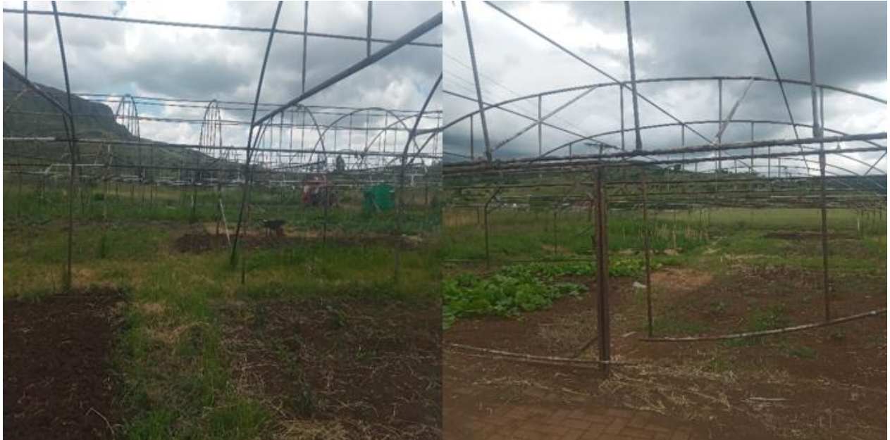
Figure 36: Greenhouse Structure for Project X in Monontsha (Fieldwork Images, 2023).
