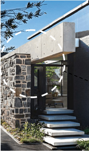
Figure 176-178: 119A Kloof stone wall with the floating planter detail (SAOTA, 2018: online) (author).
