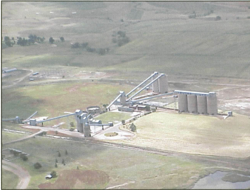
Figure 4-2. Aerial photograph of Ermelo Colliery coal processing area after rehabilitation (Photo: Chris Naudé - Ingwe Coal).
