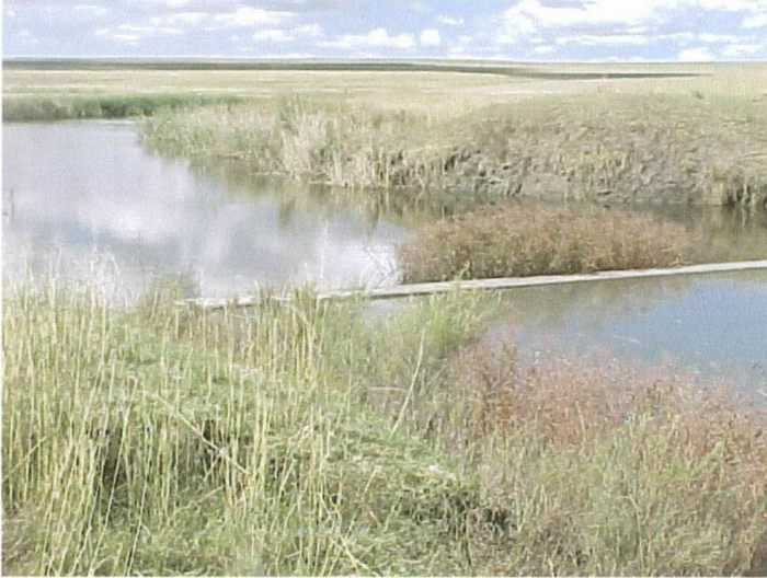
Figure 5-39. Weir at the outflow of McAlpine Lake.
