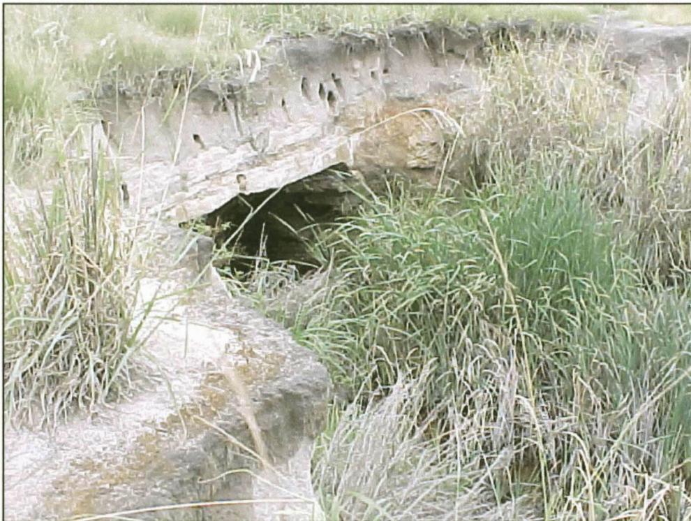
Figure 7-17. The decant position next to Dam 1.
