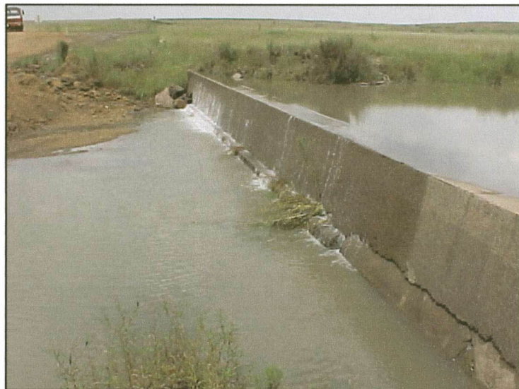
Figure 5-40. Weir in the Olifants River (January 2003).
