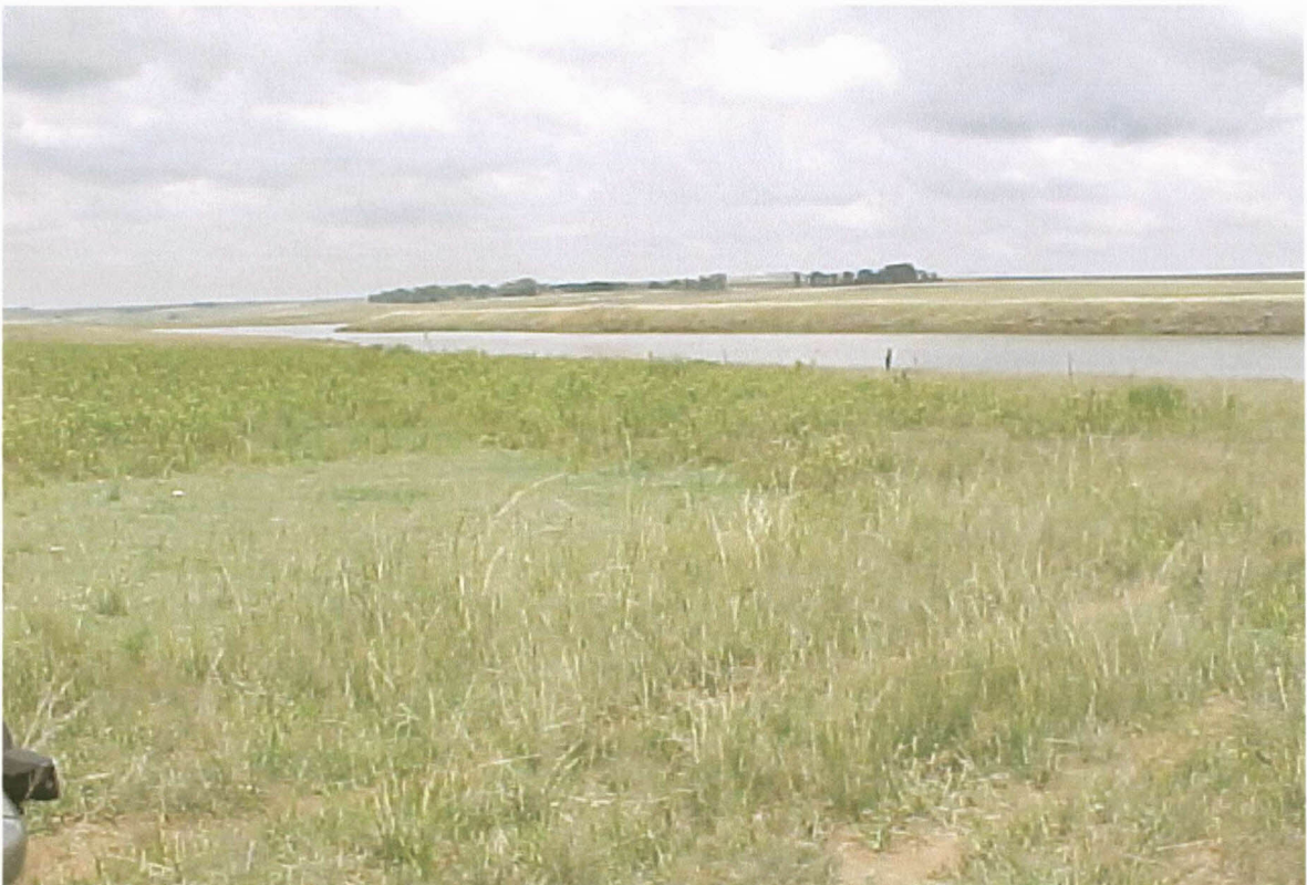
Figure 5-32. Block H Dam, adjacent to Block H Opencast.
