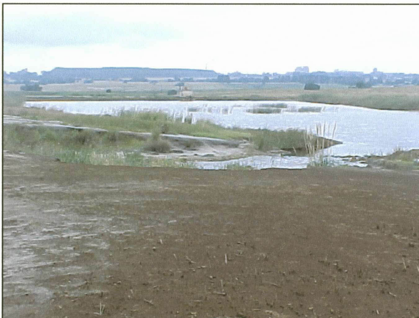
Figure 7-3. Photograph of Dam 1, with the decant point in the foreground.
