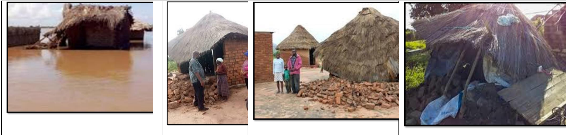
Plate P.3: Pictures of Destroyed Structures by Cyclone Idai (UNICEF, 2019)
