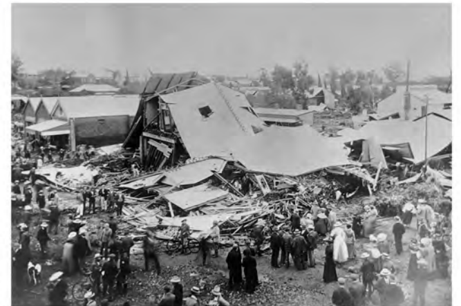
Figure 3.5: Damage done to buildings by the flood, (Collection of the National Museum, Reference number VA1721)
