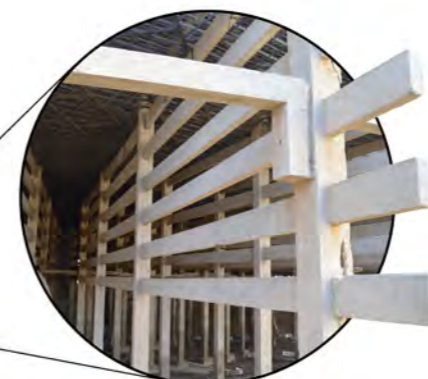
Figure 3.110: Existing internal structure, (Author, 2020)
