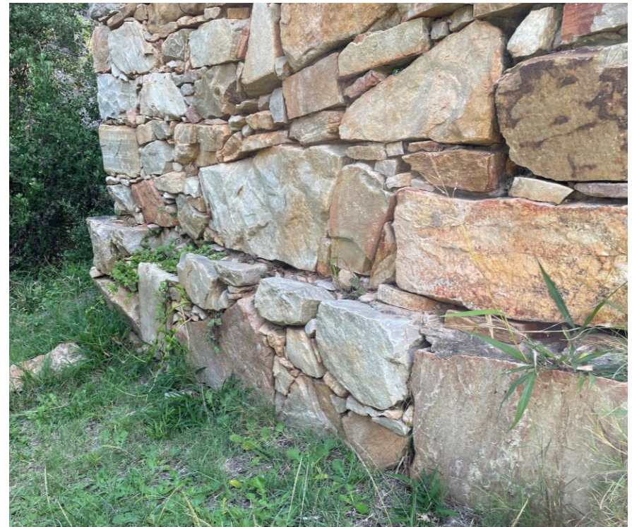
Figure 150: Existing Dry Stacked Stone Wall (Author)
