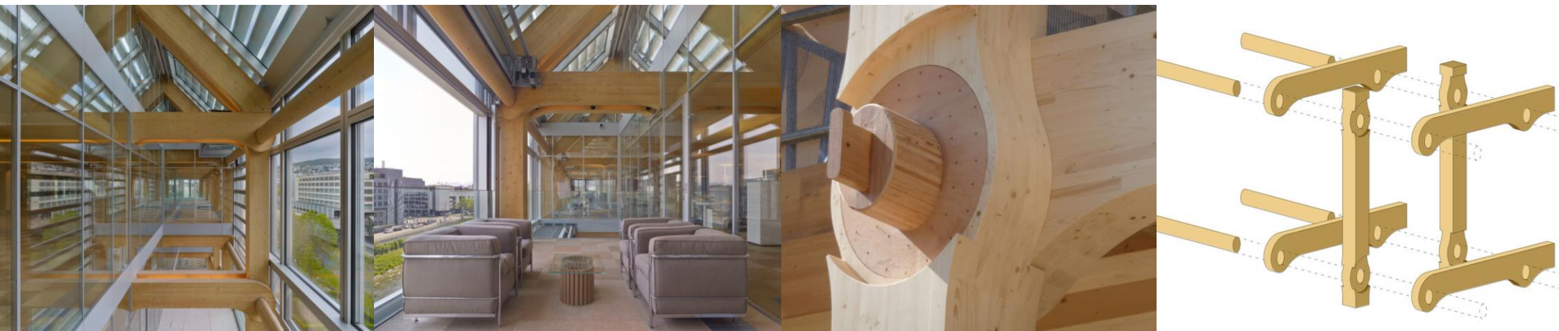
Figure 54-57: Applied Joinery in Tamedia Offices (Archdaily, 2014: online)
