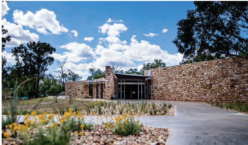
Fig. 115. Warrumbugle National Park approach to main entrance
