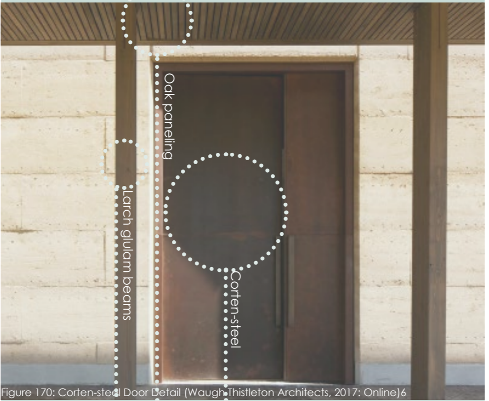
Figure 170: Corten-steel Door Detail (Wagh-Thistleton Architects, 2017: Online)6
