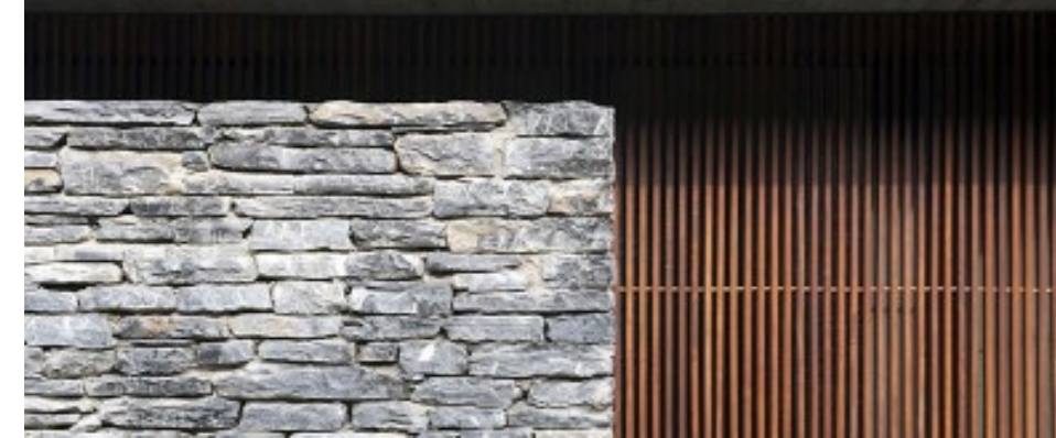
Figure 193: Sancaklar Mosque Exterior Materiality (Mayer, 2014a: Online).
