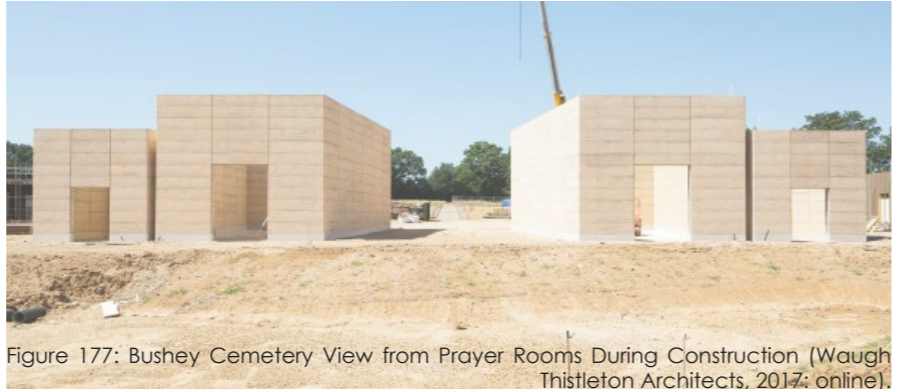
Figure 177: Bushey Cemetery View from Prayer Rooms During Construction (Waugh Thistleton Architects, 2017: online).
