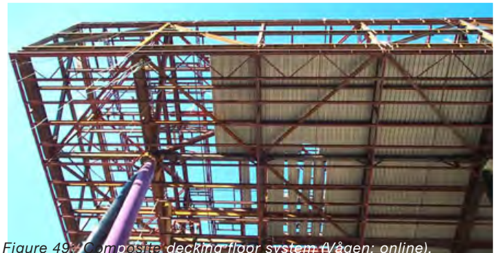
Figure 49: Composite decking floor system (Vågen: online).
