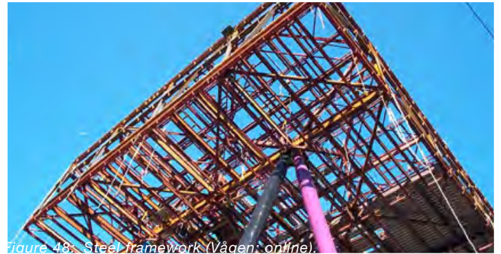
Figure 48: Steel framework (Vågen: online).
