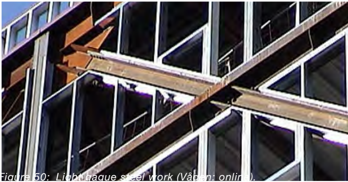
Figure 50: Light gauge steel work (Vågen: online).
