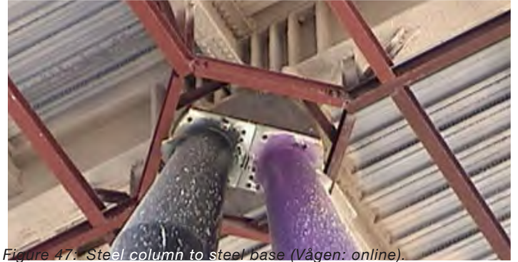
Figure 47: Steel column to steel base (Vågen: online).
