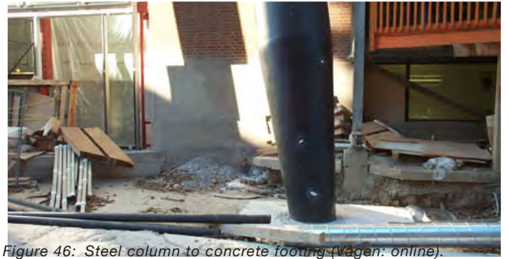
Figure 46: Steel column to concrete footing (Vågen: online).
