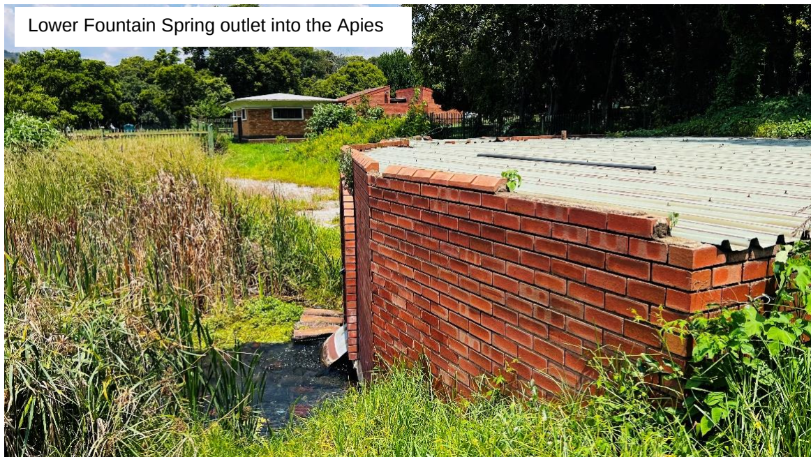
Figure 4-9: Photograph of the Lower Fountain Spring Outlet into the Apies River
