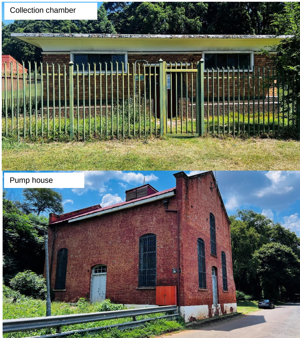
Figure 4-10: Photographs of the collection chamber and pump house receiving water from the Lower and Upper Fountain Springs
