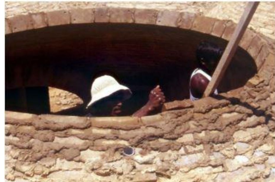
Figure.130: Checking blocks with a compass (Auroville Institute)
