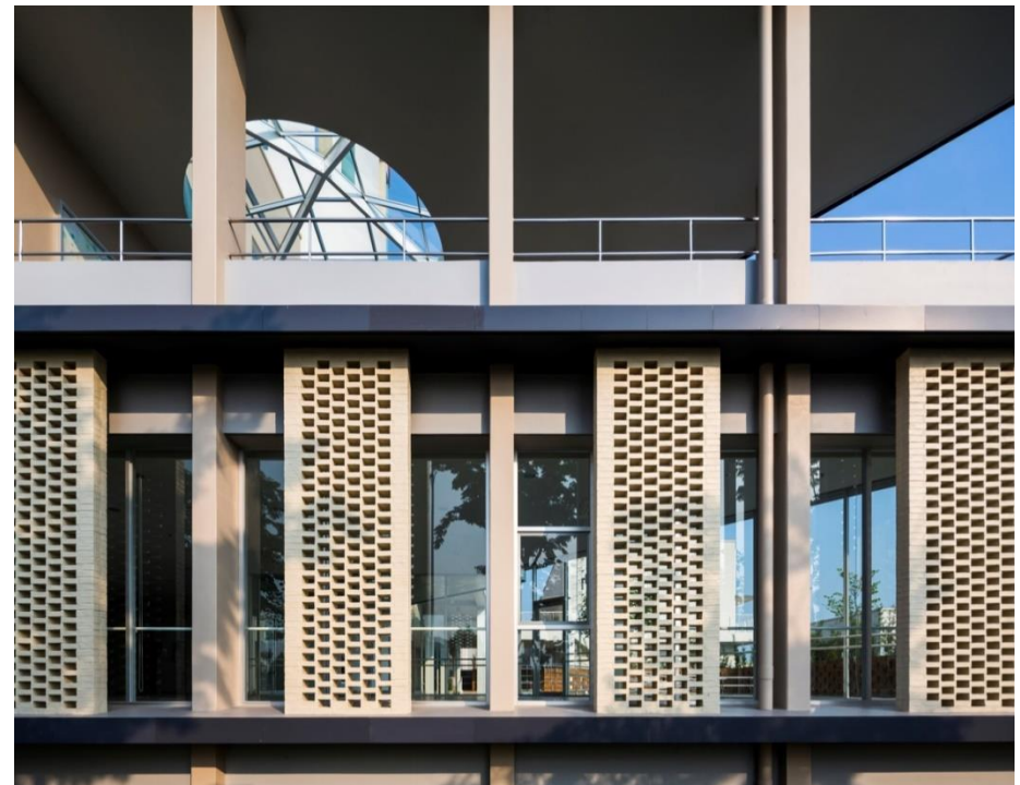
Figure 5.8; A façade which improves thermal comfort through perforated brick walls (Taisei design, 2017: Online).
