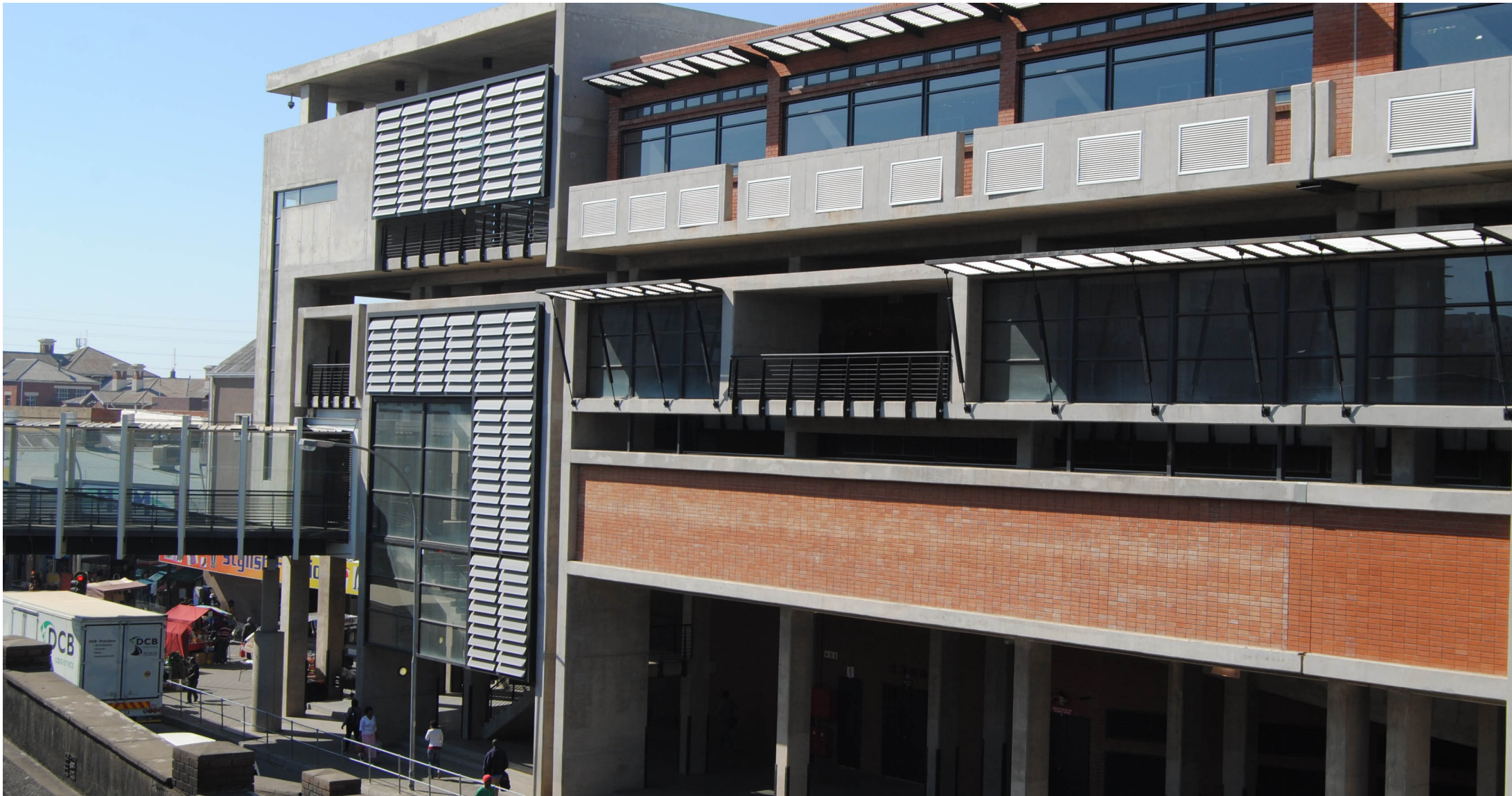
Figure 46. Mangaung Intermodal Transport Interchange (Molebatsi, T. 2013: online)
