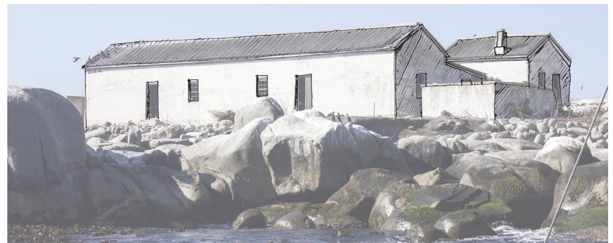
Fig 2,102 Two of the more prominent existing buildings on the site
