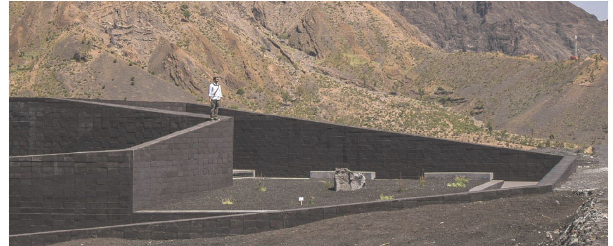
Fig 2,47 The building's exterior (OTO, 2014: online)
