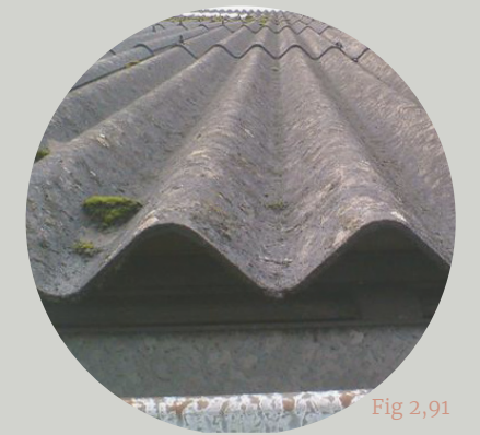
Weathered Fibre-Cement
