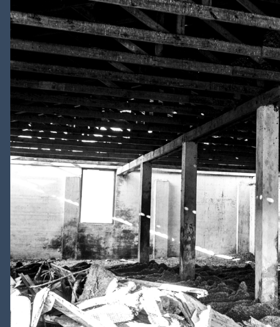
Fig 1,8 Inside an existing structure
