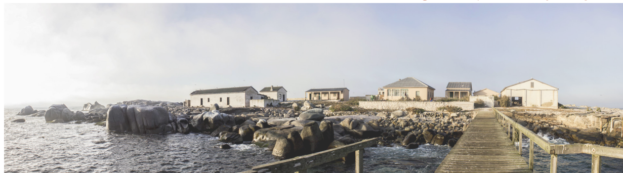
Fig 0,8 Current state of the existing structures
