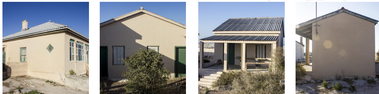
Fig 3,79 Photographs of the proposed demolished structures
