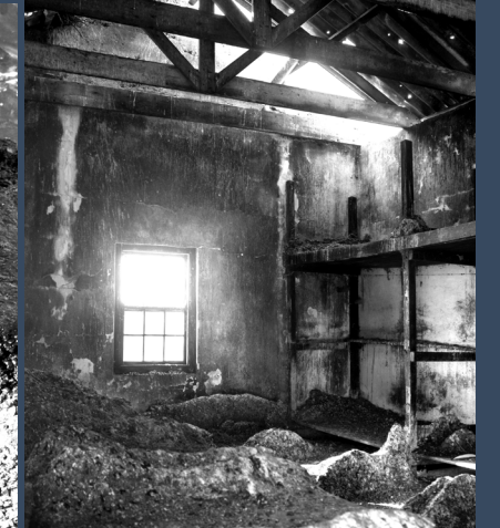
Fig 1,10 Inside an existing structure
