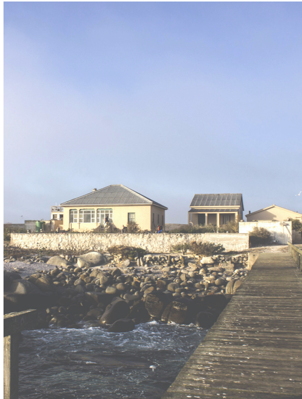
Fig 3,98 View from the jetty
