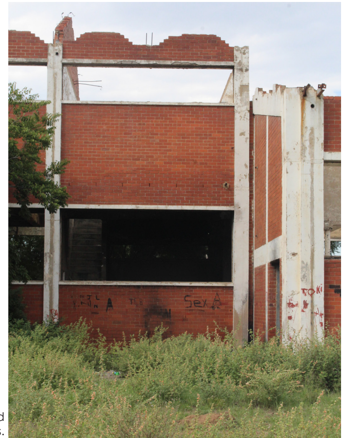
Fig. 88. Brick infill and concrete columns.
