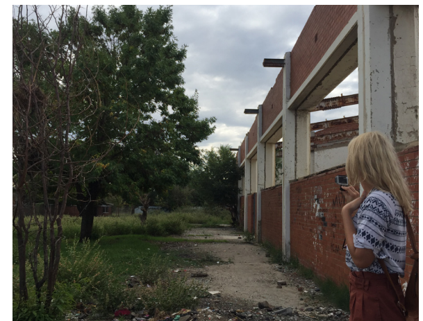
Fig 362. Photo of the inside of existing portal frame building
