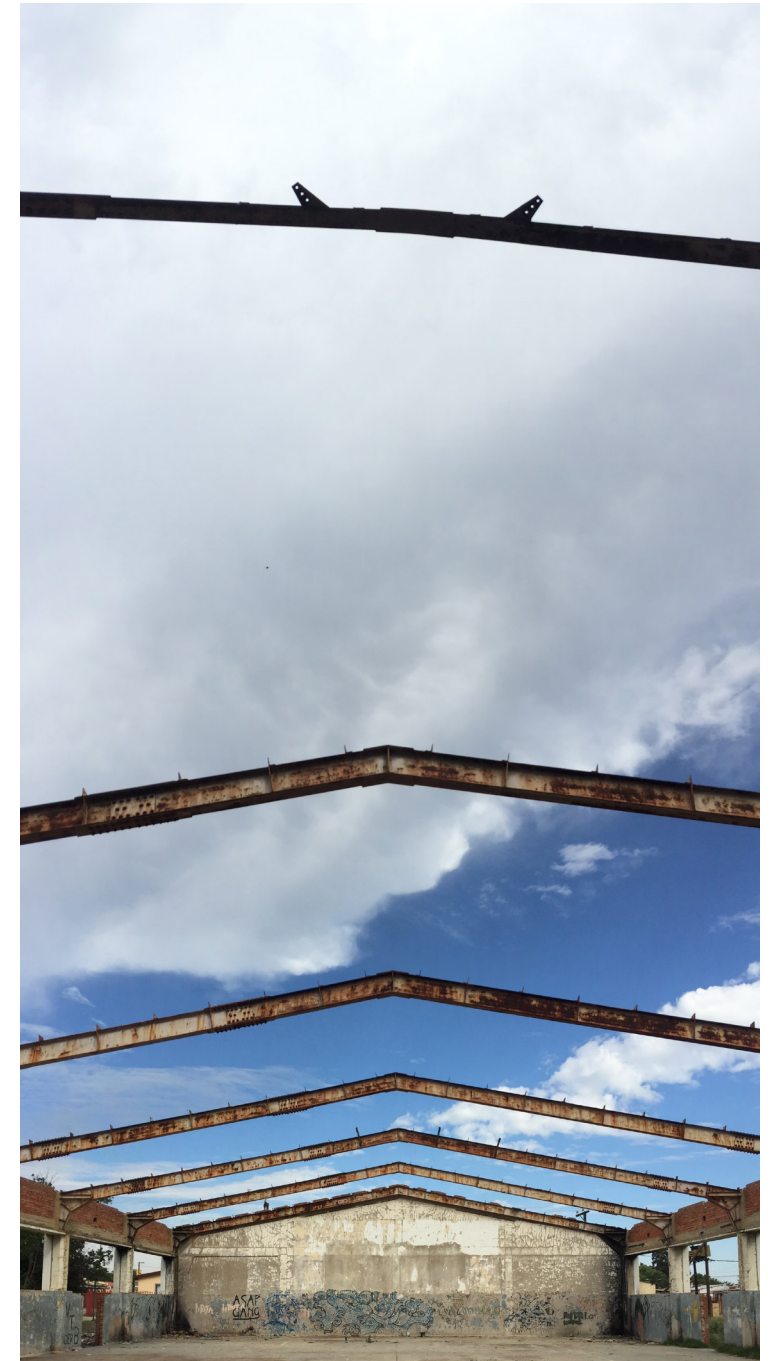
Fig. 81. Existing roof structure.
