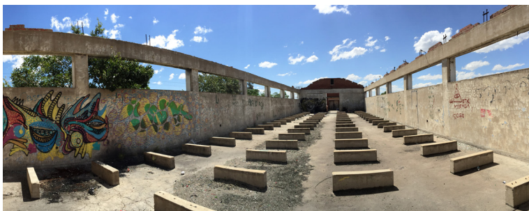
Fig 87. Second floor with no existing roof or roof structure.
