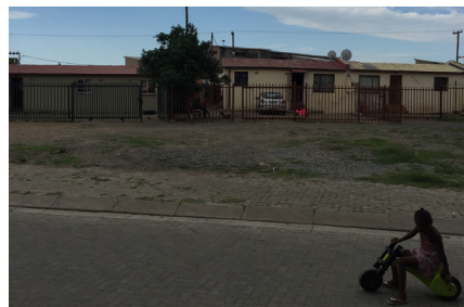
Fig. 80. View of Batho houses as seen from site.
