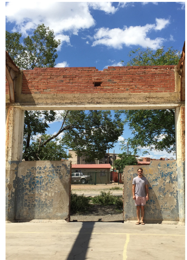
Fig 361. Photo of the inside of existing portal frame building
