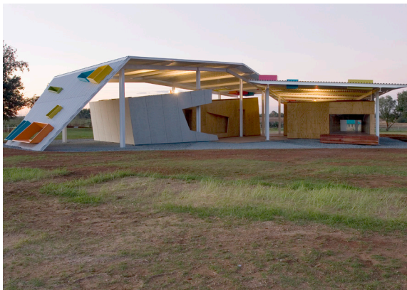
Fig. 18. View of Olifantsvlei Primary School
