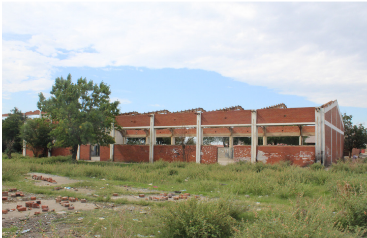
Fig. 82. Brick infill
