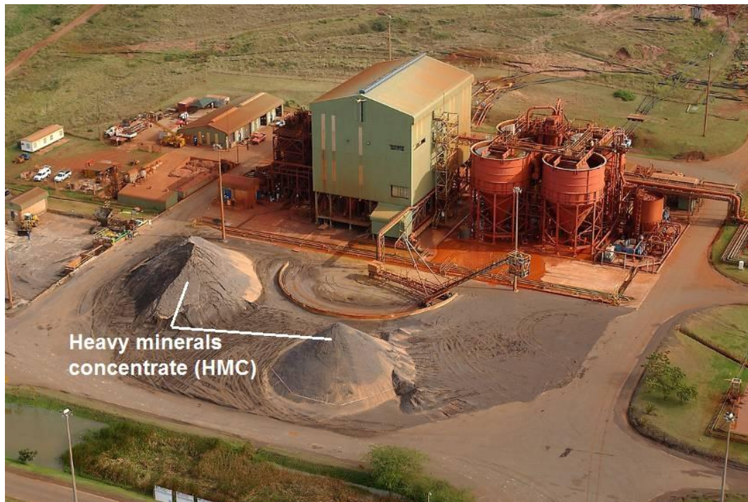
Figure 2.4: A photograph of the primary wet plant (PWP) with non- and low magnetic heavy minerals concentrate (HMC) seen in the foreground. This material is transported by truck to the central processing plant (CPC) near Empangeni for further processing.
