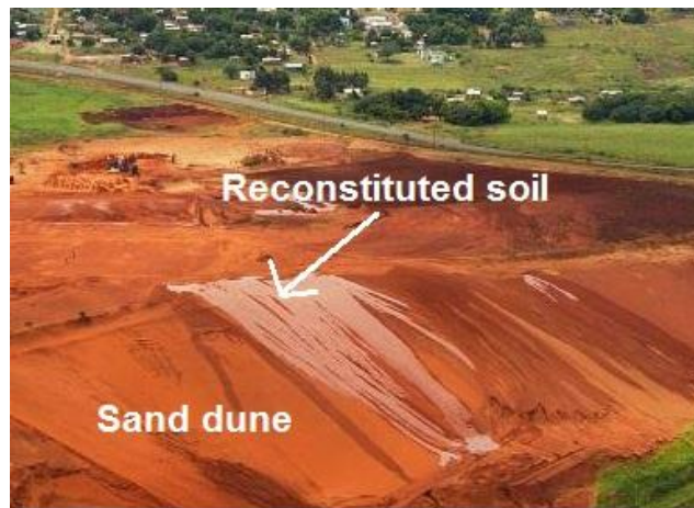
Figure 2.6: A reconstructed sand dune being covered with reconstituted soil.
