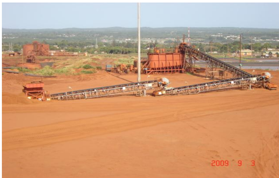
Figure 2.7: A photograph of the bulk mixing plant (BMP). Sand is being fed on a conveyer belt into the plant where it is mixed with slimes. The resultant mixture is known as the reconstituted soil.
