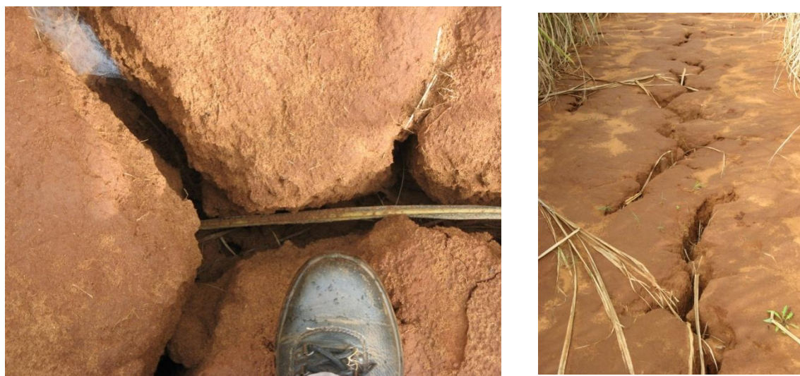
Figure 3.8: Photographs showing deep cracks in the reconstituted soil.
