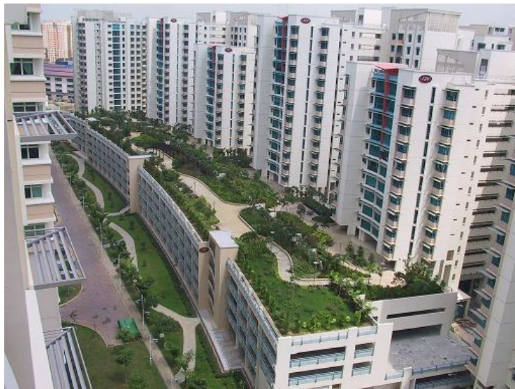
Figure 2.6: An example of an intensive green rooftop system.
