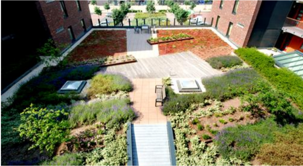
Figure 2.4: An example of a semi-intensive rooftop system.
