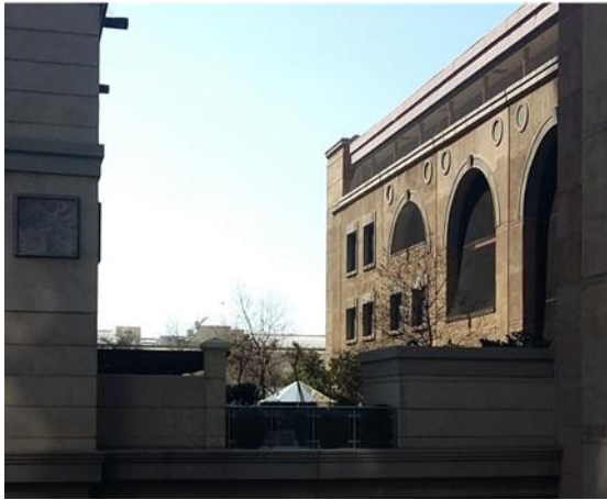
Figure 7.4: Green rooftop system on The Michealangelo hotel
