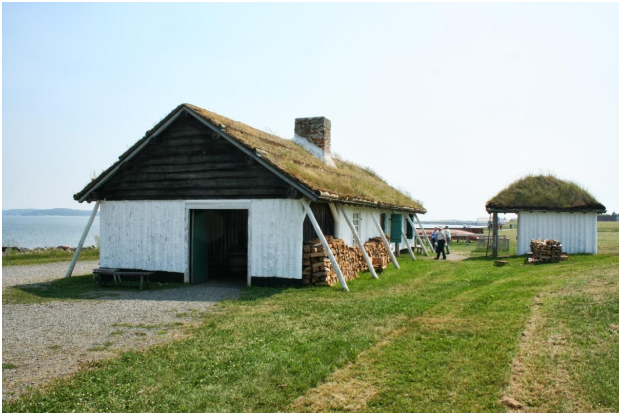
Figure 2.2: An example of an extensive rooftop system.
