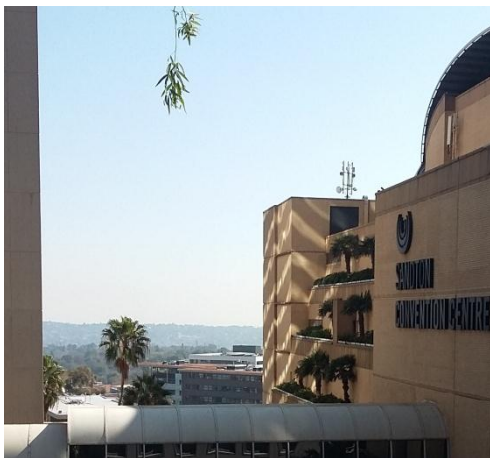
Figure 7.5: Green rooftop system on the Sandton Convention Centre
