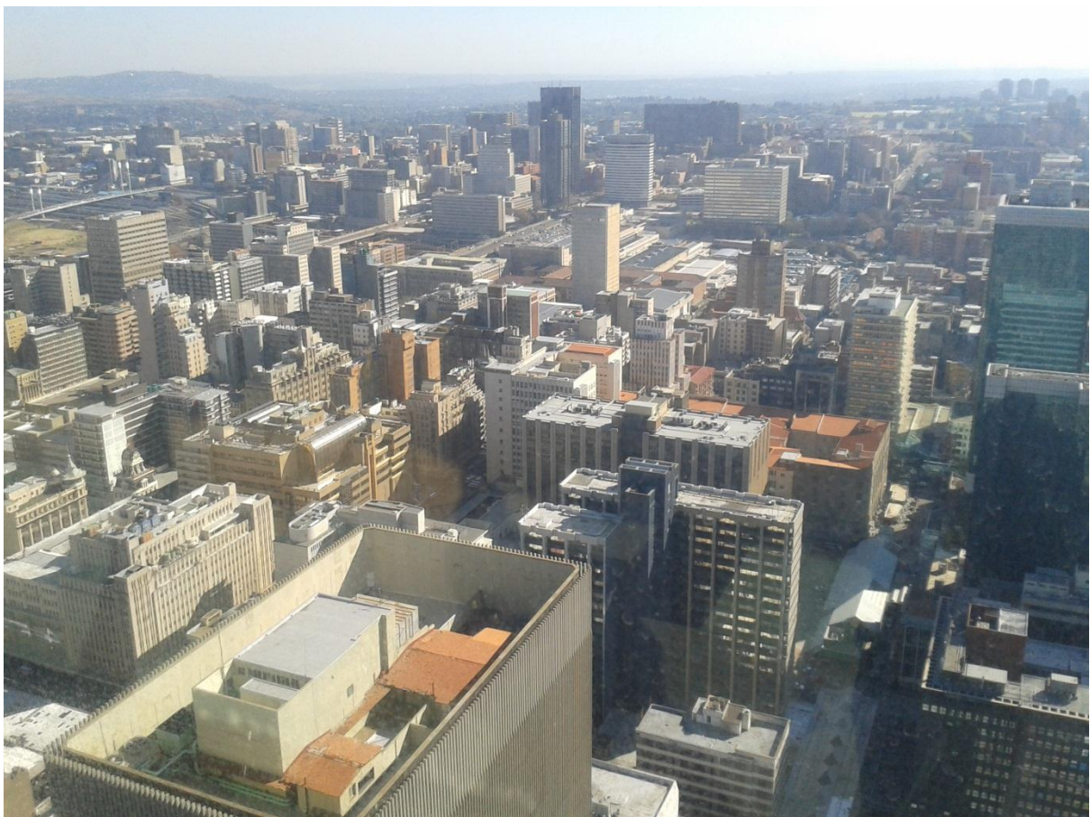
Figure 7.1: Roofs of buildings in Johannesburg CBD
