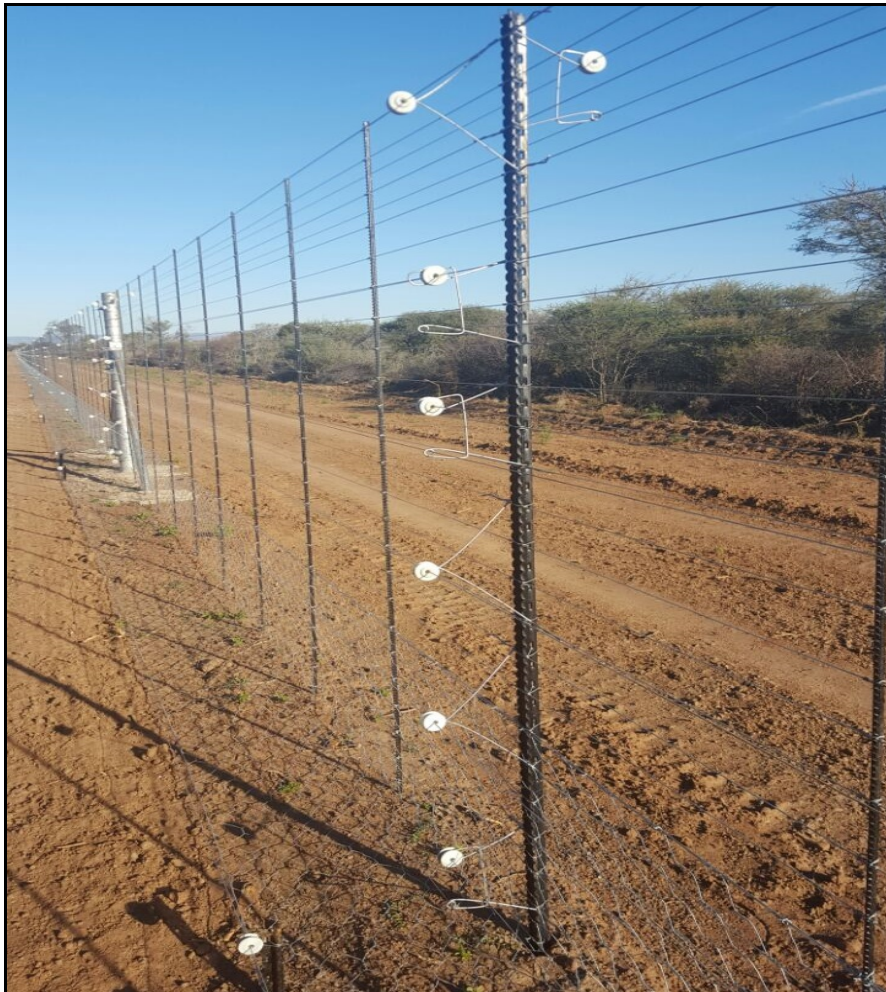
Slide 2.1. The electrified perimeter wildlife fence of the Reserve.
