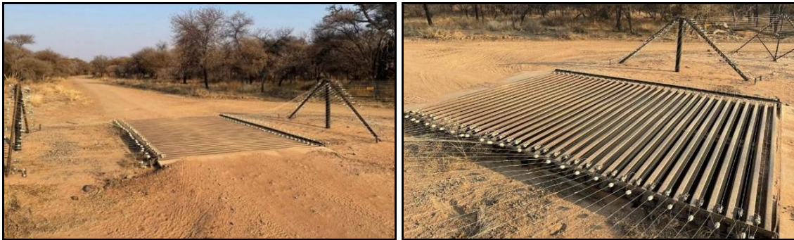
Slides 4.36 & 4.37. The custom steel cattlegrid gate used to keep dangerous wildlife from entering the safe area where staff is housed on the Reserve.
