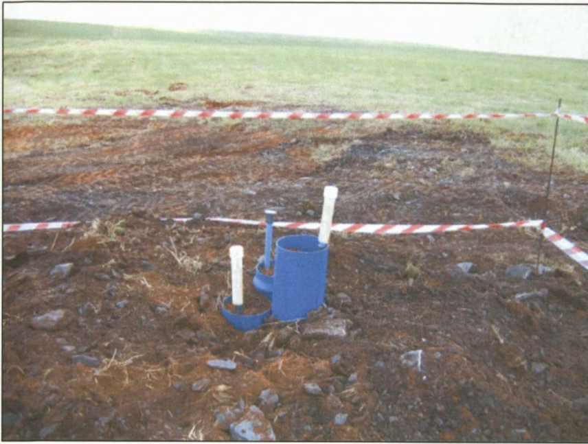
Figure 7-40: Installed leaching columns at Optimum pivot.
