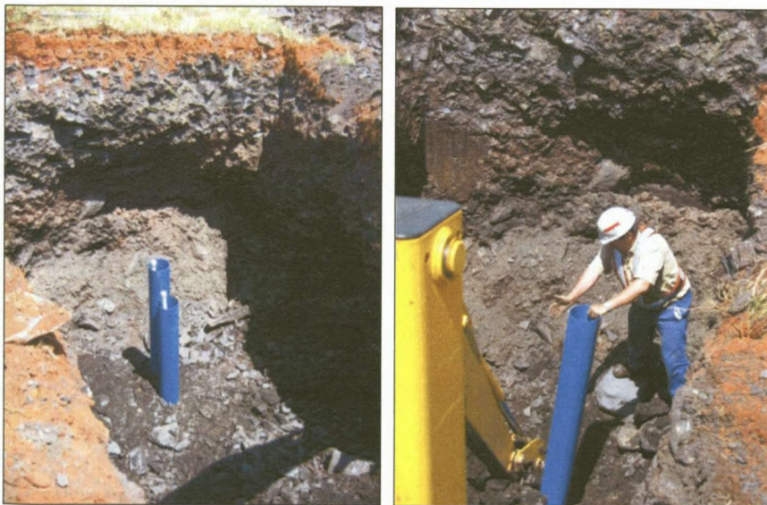
Figure 7-39: Installation of leaching columns.
