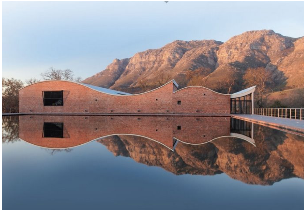
Fig.52: Dornier main facade reflected over water roof (Dornier, 2022: Online).
