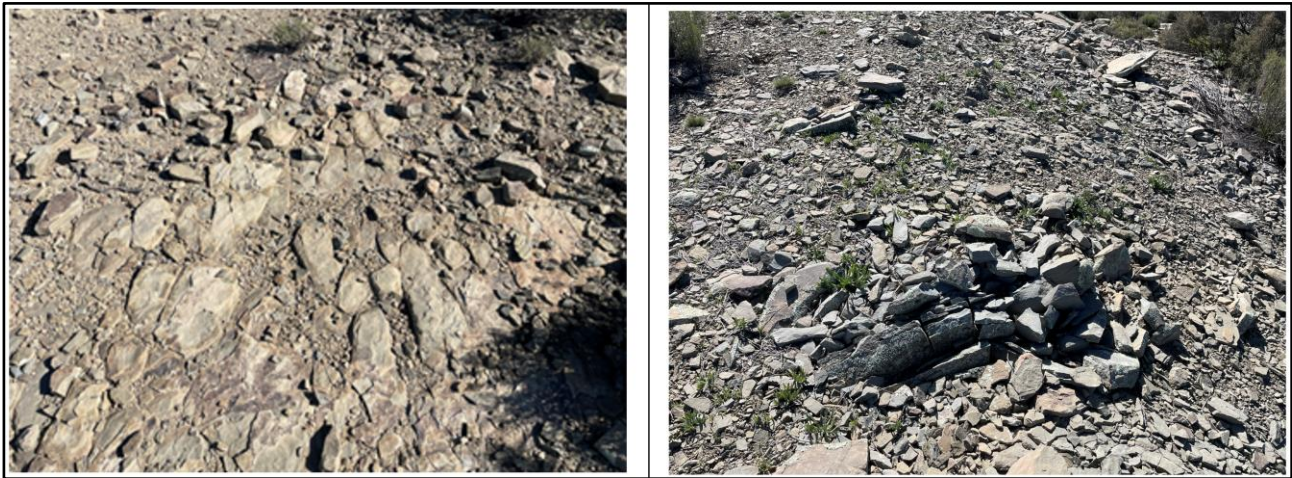
Figure 25: Fractured sandstone outcrop in a depression associated with major structure F3 (-32.446615°S, 20.619237°E) (Authors own)
