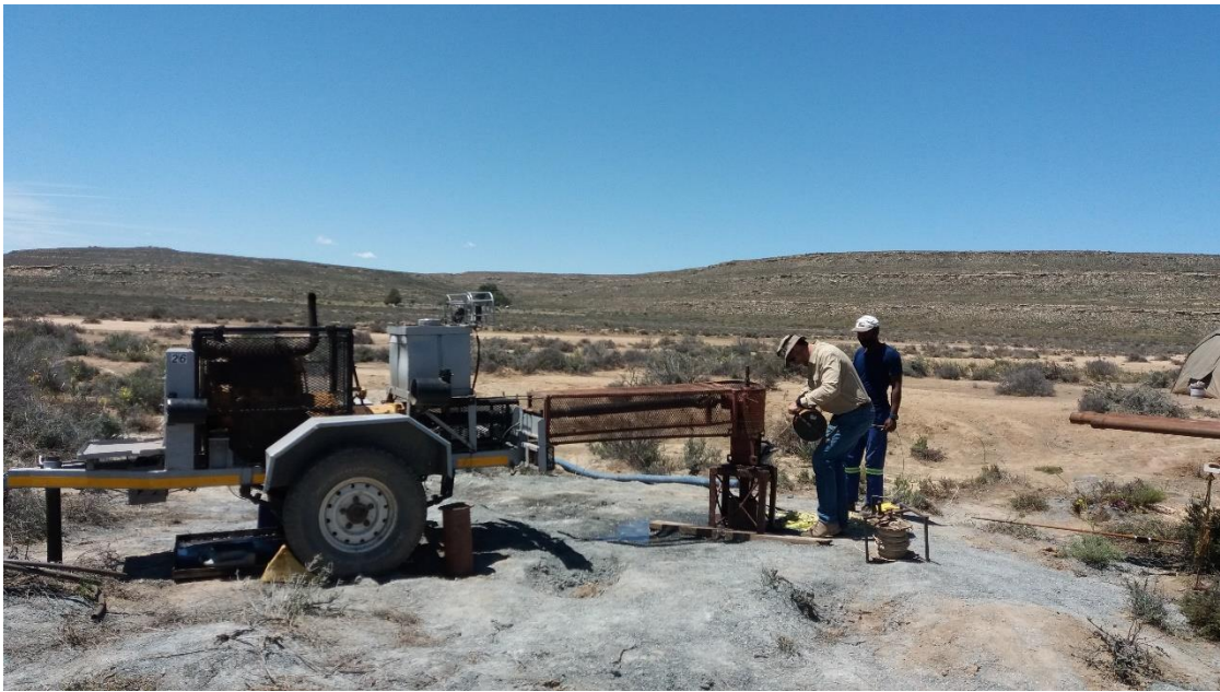
Figure 46: Pumping test at SL3 (author's own)
