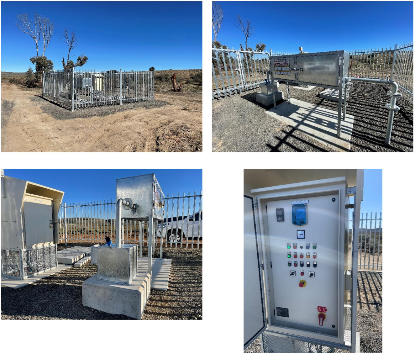
Figure 74: Wellhead protection at SL 11 with a fenced zone around the production hole and associated headworks
