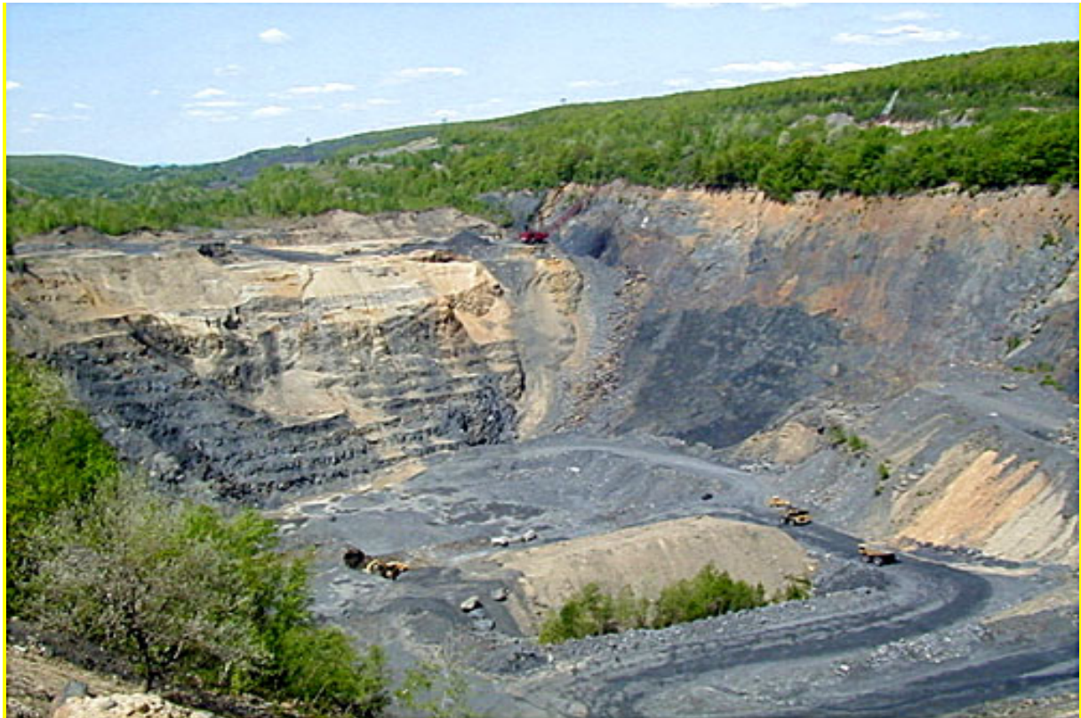
Figure 3: Open-pit mining (www.numahammers.com)
