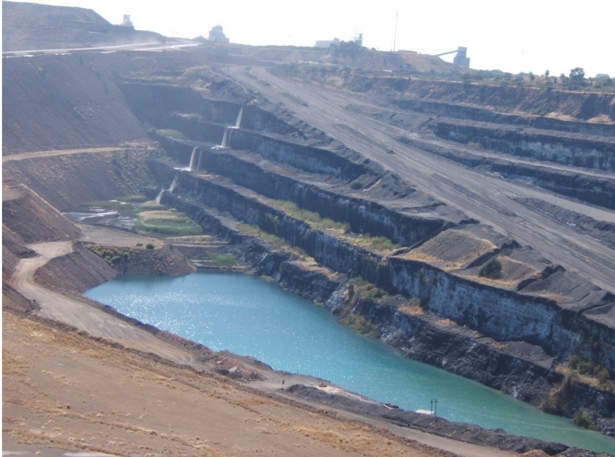
Figure 159: An obsolete sump being backfilled, courtesy of the Grootegeluk mine.
