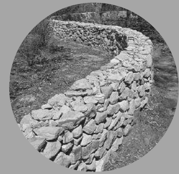
Figure 107 &108: Dry-stacked Sandstone wall and local application in Korannaberg (Author)
