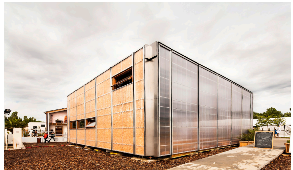
Figure 83: Resso house south facade filled with strawbale for heat insulation (Archdaily, 2015: online)
