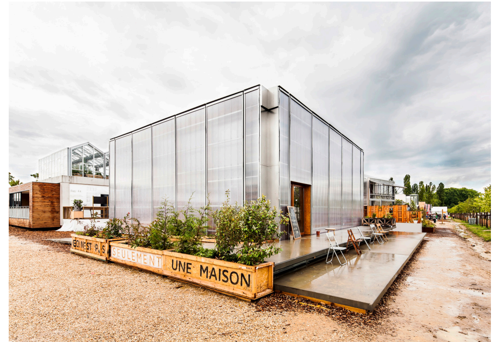
Figure 90: Polycarbonate facade Resso House (Archdaily, 2015:online)
