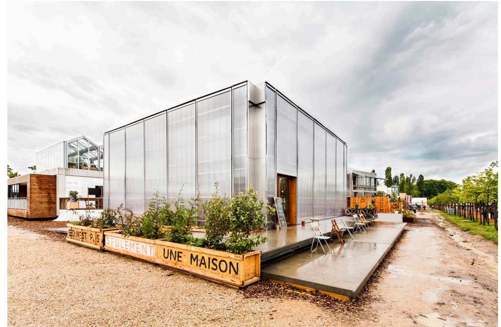
Figure 82: Resso house Polycarbonate clad exterior (Archdaily, 2015: online)
