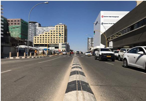
Figure 62: Independence Avenue Buildings adjacent to site (Author, 2019)
