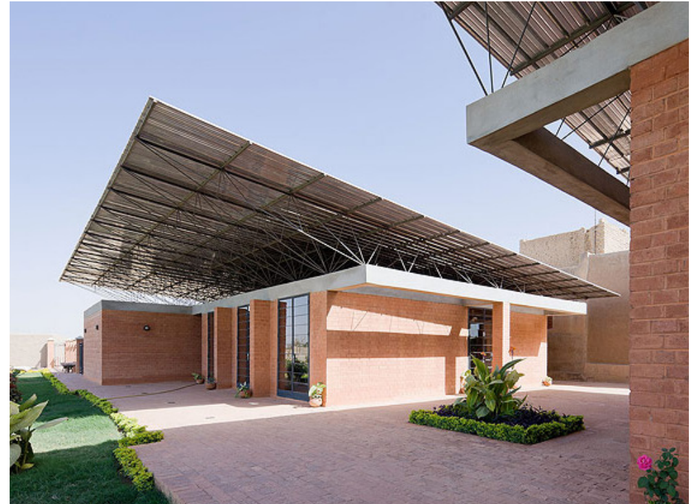
Figure 78: Large overhangs shade and keep walls cool, ensuring well controlled interior spaces (Archdaily, 2010:online)
