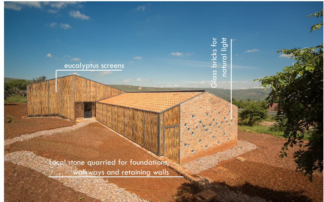
Figure 73: Natural low cost material building envelope (Archdaily, 2016:online)
