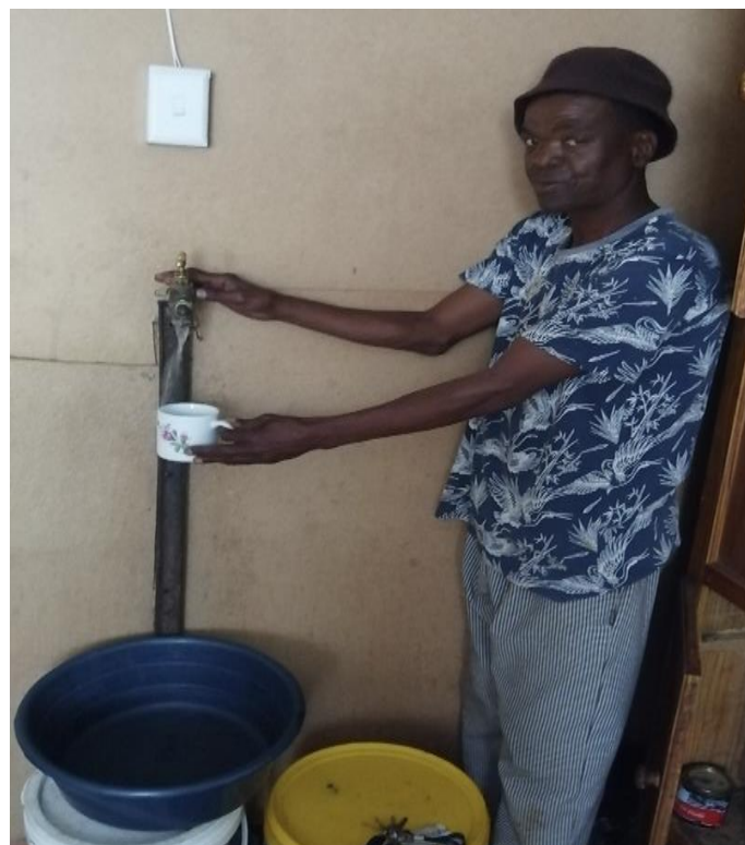
Figure 6.11: Illegal connection of water from the communal standpipe to the house
